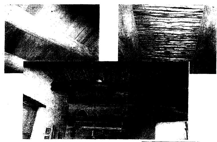
PLEASE NOTE...that our vigas and latillas are the real thing. They are natural whole trees changed only by the peeling of the bark, and are not perfect. As drying of the wood occurs in our Arizona climate, checking and shrinking will occur. Unlike machined "peeler poles", our vigas have character, knots and dryness checking. We assure you that Old Pueblo's vigas and latillas will offer an authentic look to your project.
