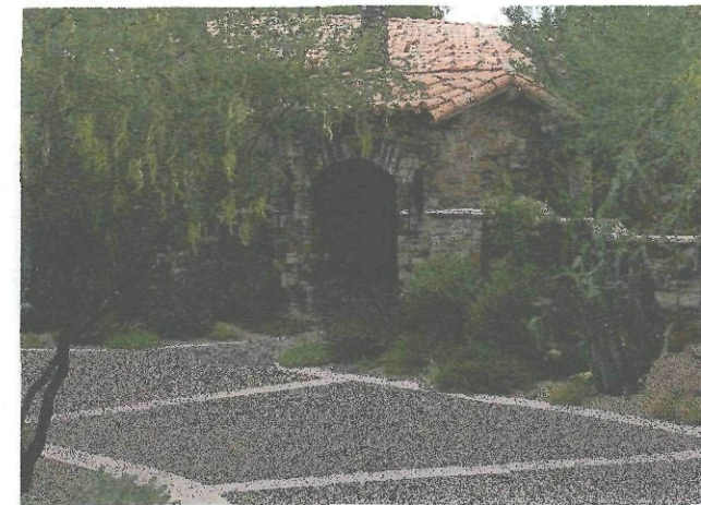
Stone / Tile Roofing / Agg. Paving with Banding
