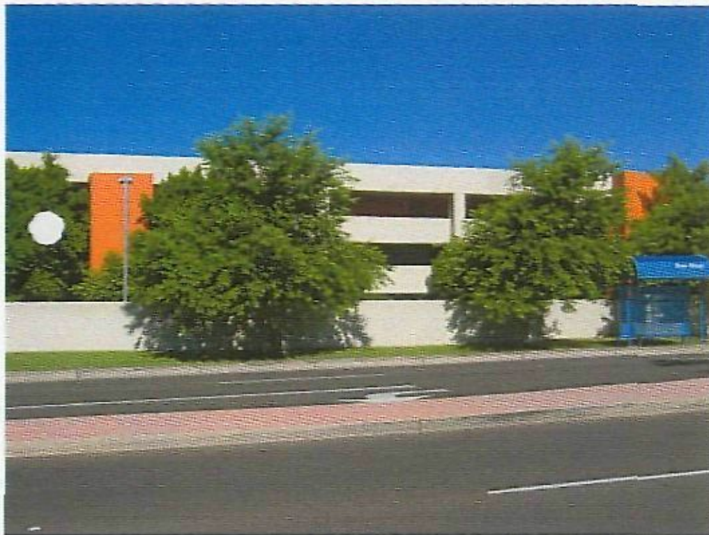
EXISTING - EAST ELEVATION DRINKWATER BLVD.
