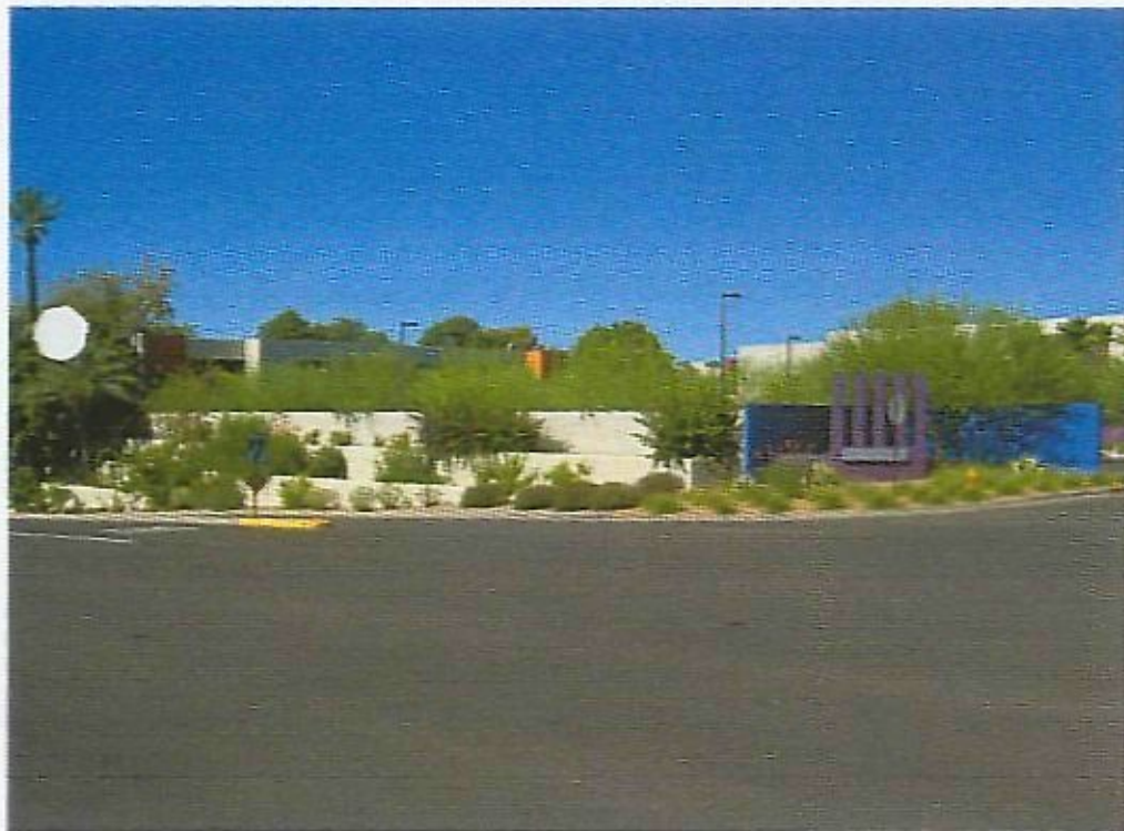
EXISTING - EAST ELEVATION DRINKWATER BLVD. ENTRANCE
