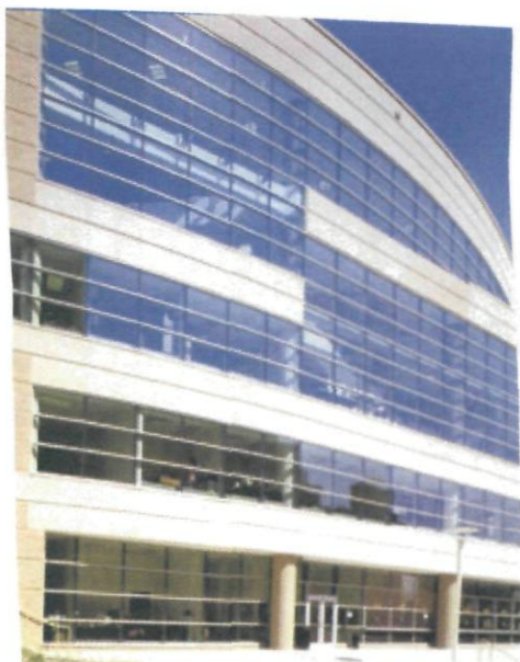
Glazing: 1" Insulated Low-E Double Pane Glass
