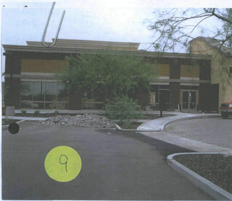
View from Rear of Building 9343 E. Shea Blvd.
