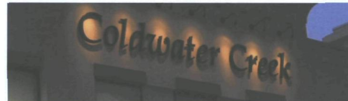
External/indirect illuminated reverse pan-channel letter.
