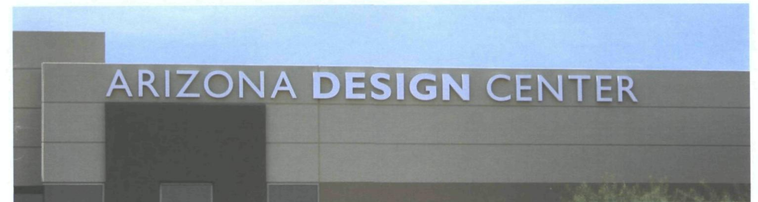
Halo illuminated reverse pan-channel letter examples.
