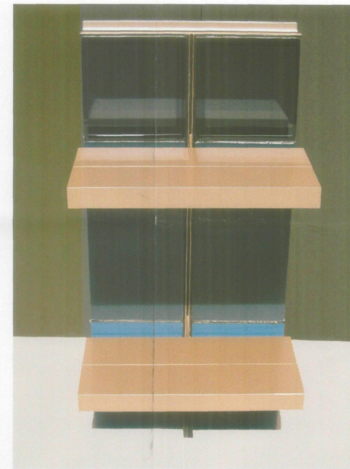
Mock-up: Window wall / Fins
