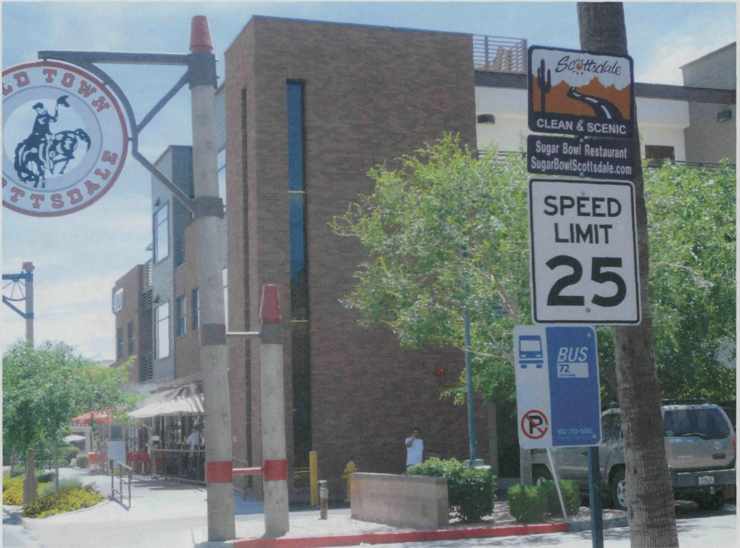
North Elevation View
