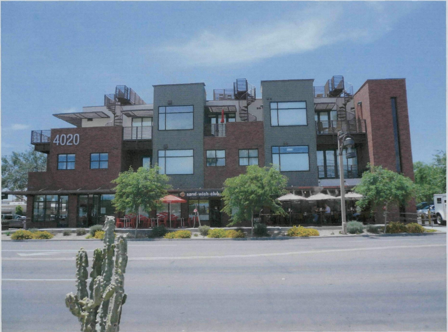
East Elevation View
