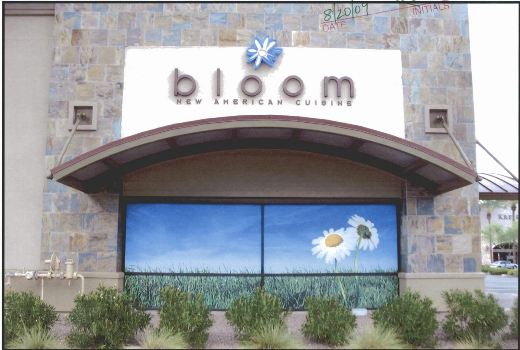
West Elevation (Close-up)
