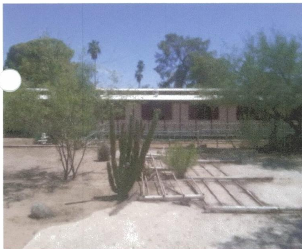
4. Looking South from Site
