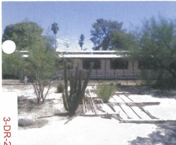
4. Looking South from Site
