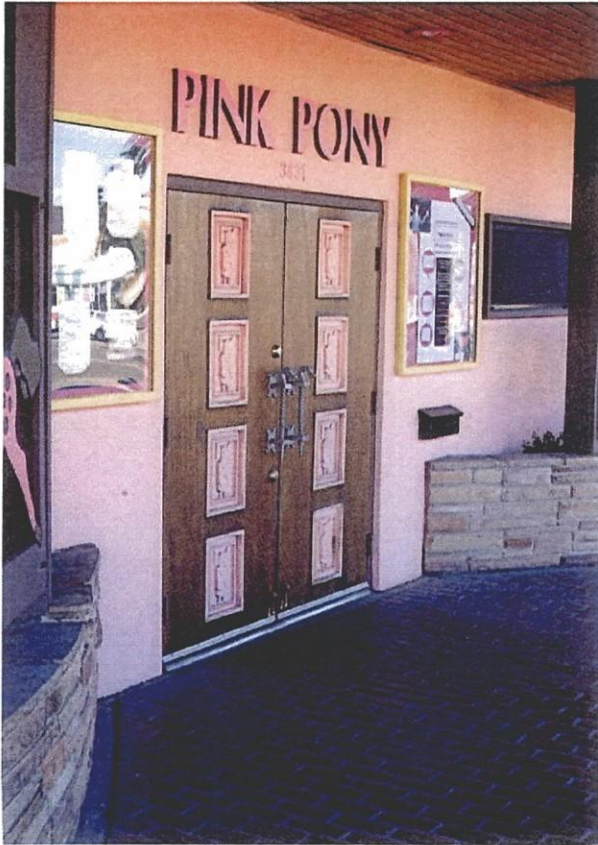
Stucco wall around recessed entry
