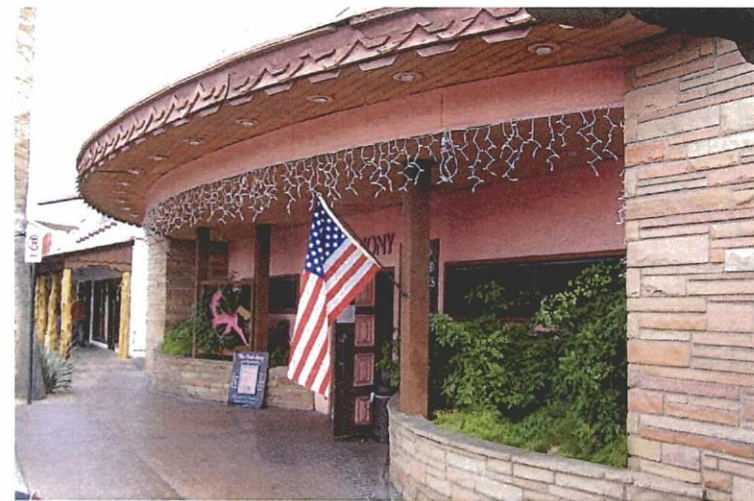
Canopy, wooden posts and horizontal windows by entry
