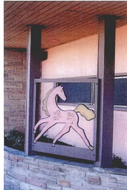
Wooden posts supporting canopy and horizontal window
