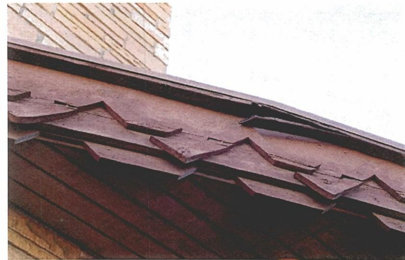
Canopy fascia and trim
