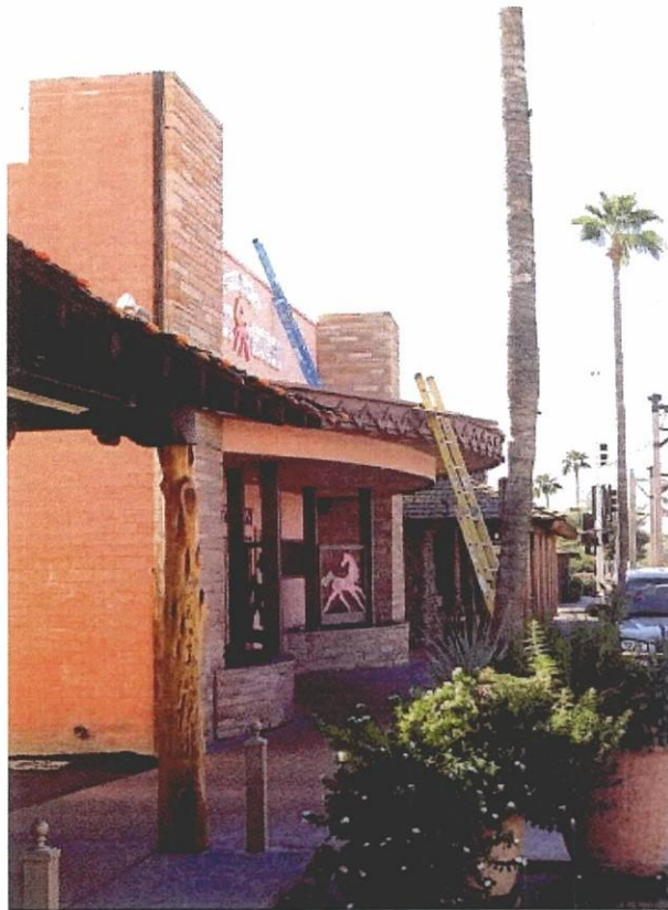
Looking south at corner elements and parapets
