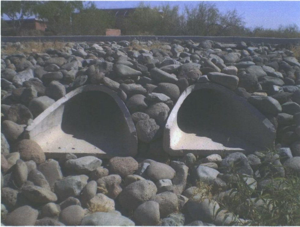
Photo 1. Culvert west of 98 th Street
