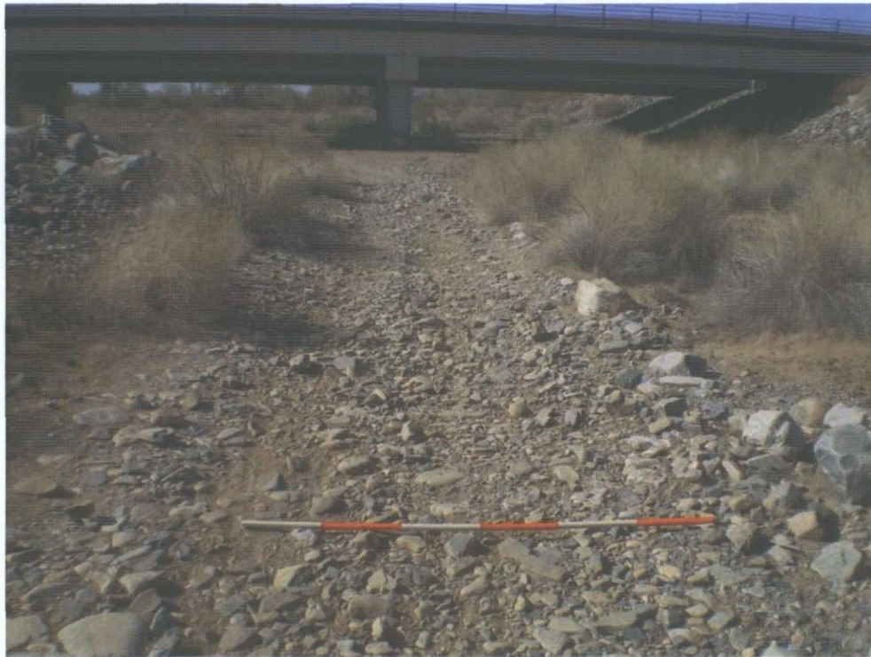
Photo 11. Upstream view of Reata Pass Wash (6 ft)
