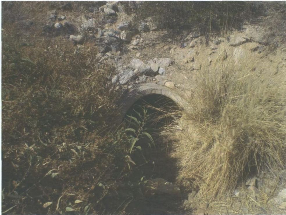
Photo 7. Culvert at 98 th Street & Bell Road
