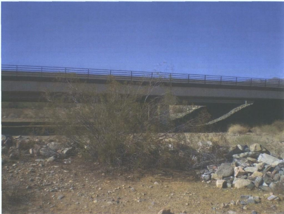
Photo 10 . View to north at Bell Road
