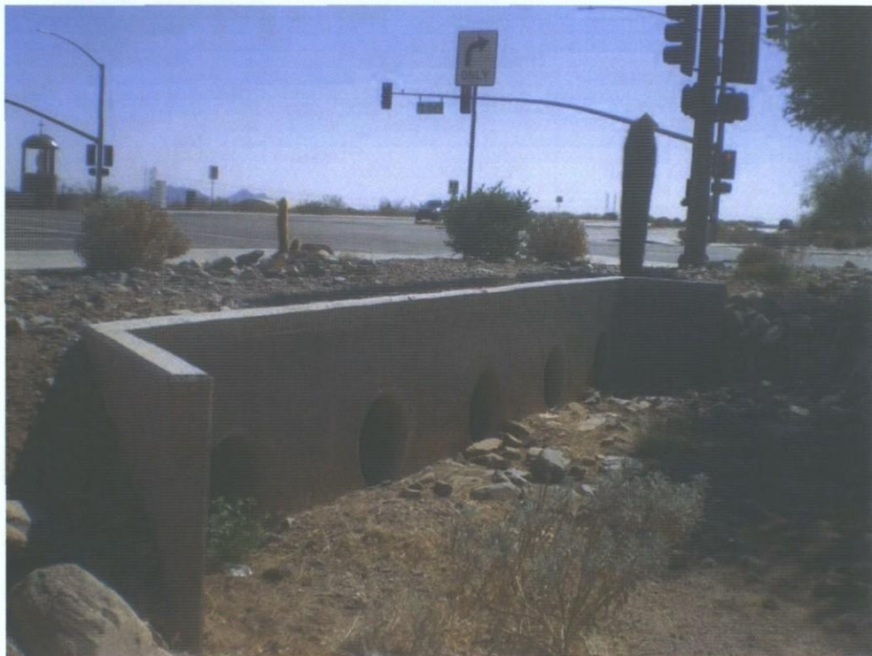
Photo 8. View southwest of culverts at Bell Road & 98 th Street intersection
