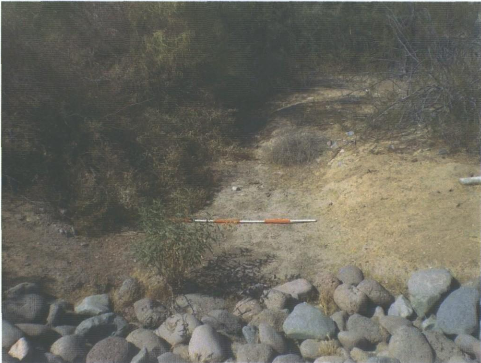
Photo 2. Upstream view at culvert west of 98 th Street (6ft)
