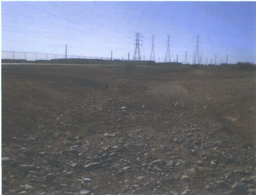
Photo 24. View to northwest of drainage channel parallel to Reata Pass Wash
