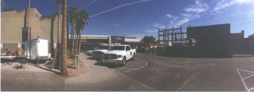
15 - SOUTHEAST CORNER LOOKING SOUTHEAST
