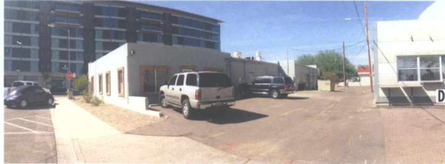
8 - NORTHWEST CORNER LOOKING NORTHEAST
