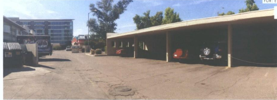
10 - NORTHEAST CORNER LOOKING NORTHWEST
