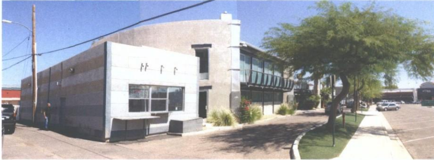
1 - SOUTHWEST CORNER LOOKING NORTHEAST
