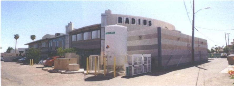
5 - NORTHWEST CORNER LOOKING SOUTHEAST
