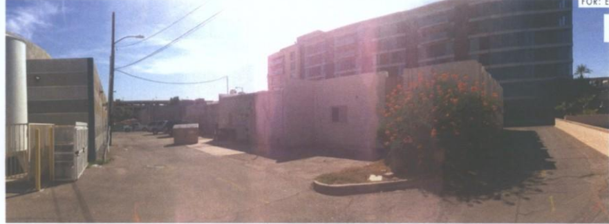
6 - NORTHWEST CORNER LOOKING SW
