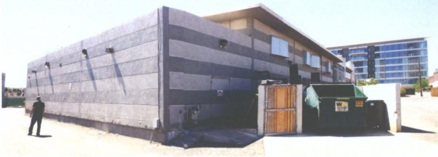
9 - NORTHEAST CORNER LOOKING SOUTHWEST
