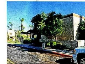
6 VIEW TO EAST/SOUTHEAST
