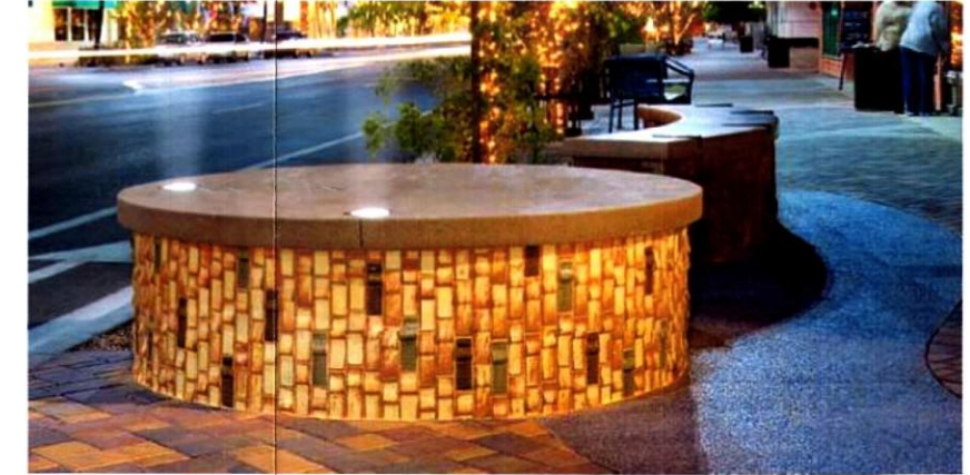
Custom Seatwalls and Art Plinths with cast-in-place cap and aesthetic exterior treatment
