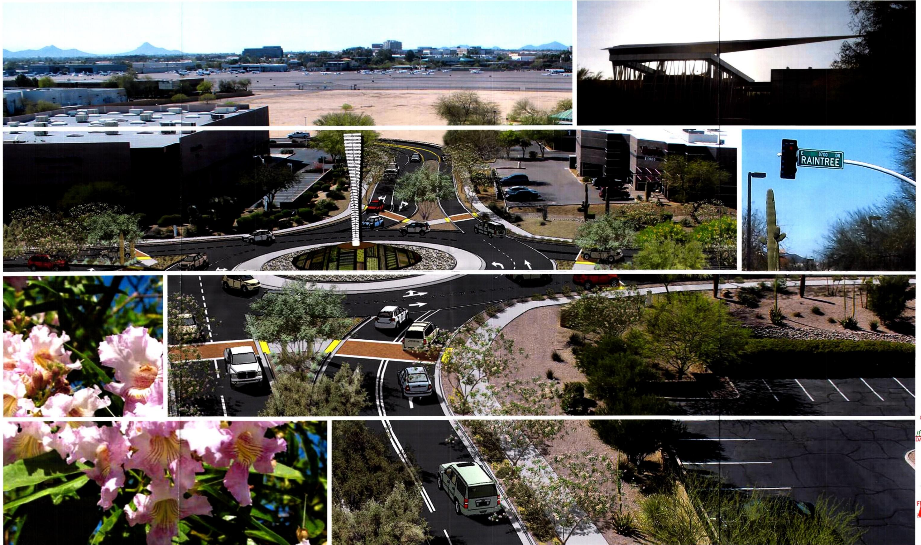
Scottsdale Road to Loop 101 Freeway
