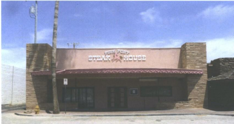
View of Front Facade
