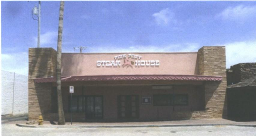
View of Front Facade
