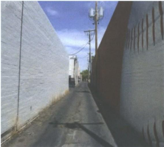
Alley & Adjacent Bldg.
