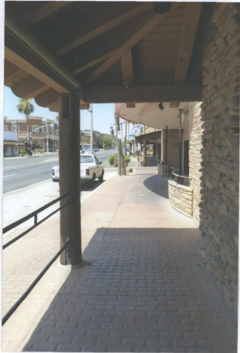
LOOKING NORTH @ BANDERAS
