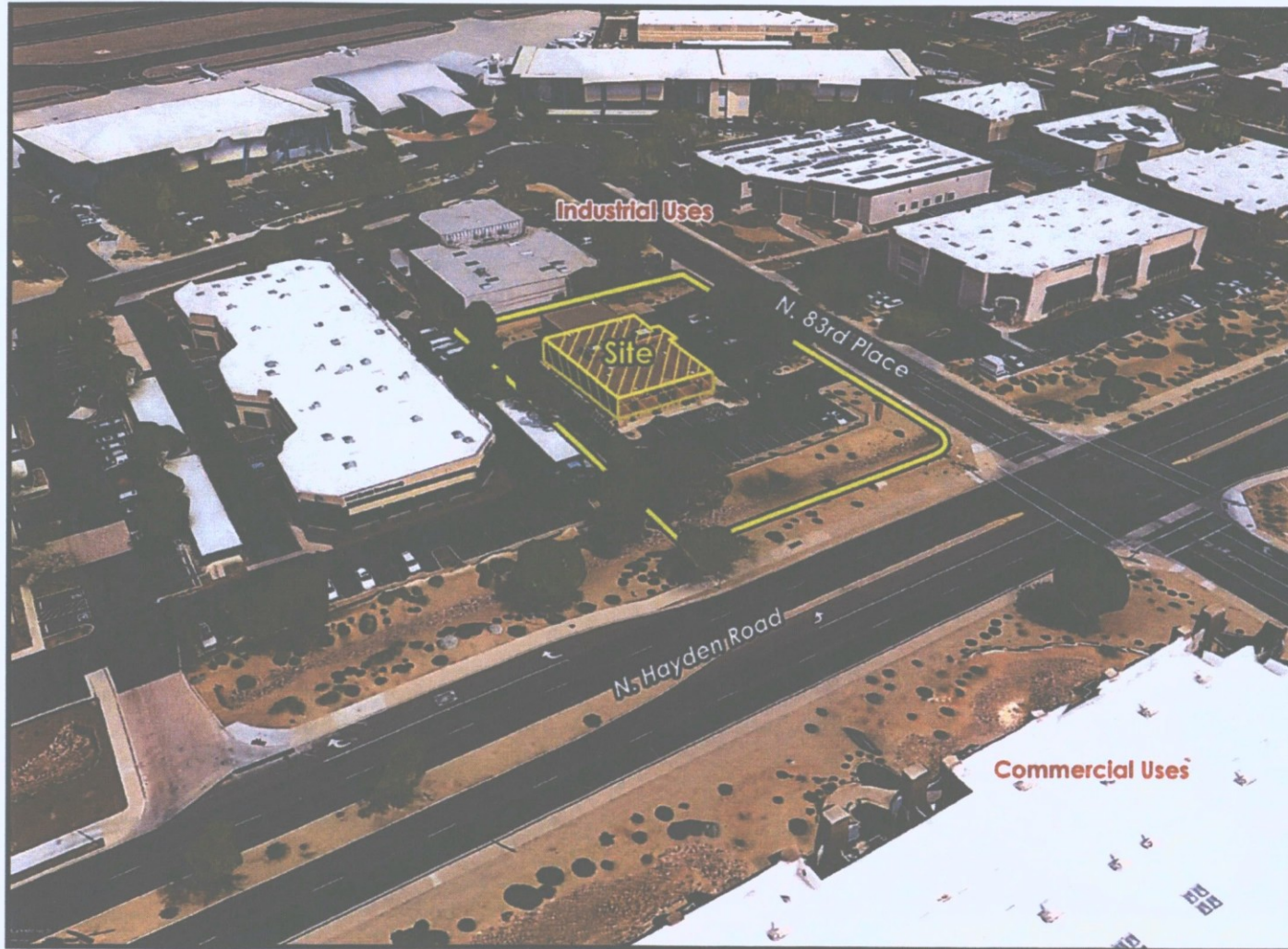
OBLIQUE DETAIL AERIAL
