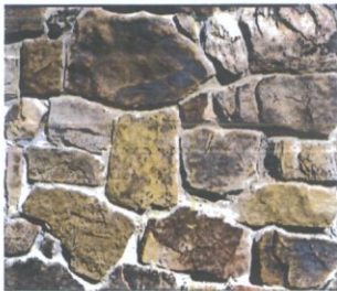
STRUCK MORTAR JOINT
