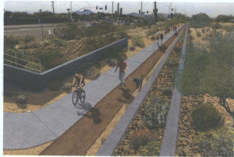
2. View looking West towards 124th St. and Shea Blvd.
