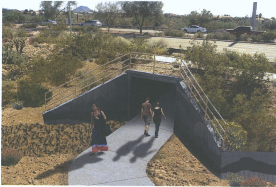
1. View looking at the North Tunnel Access under Shea Blvd.
