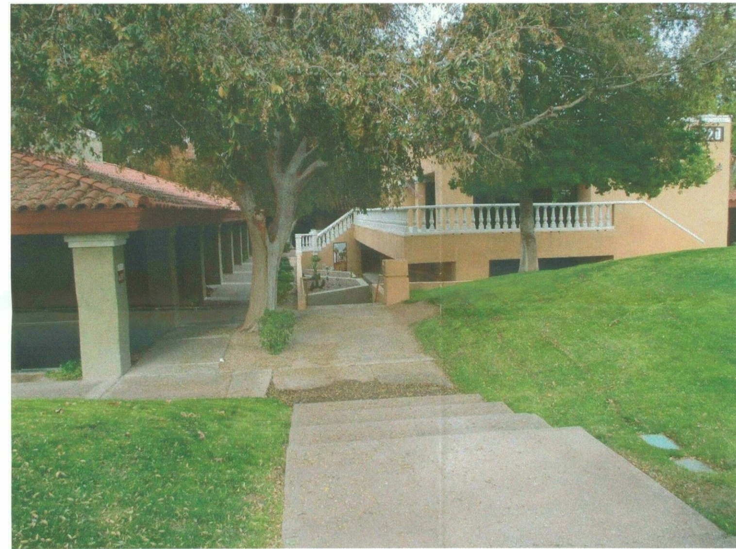
VIEW J - BLDG 6320
