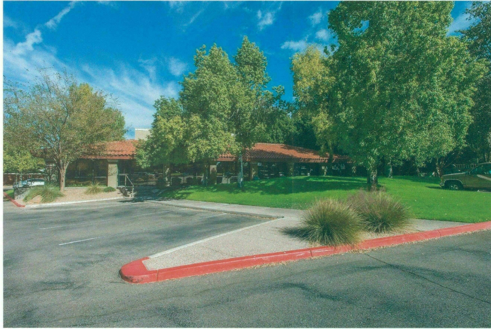
VIEW H - BLDG 6320 + LAWN
