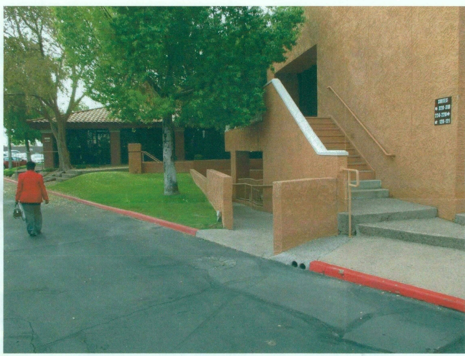
VIEW L - BLDG 6350
