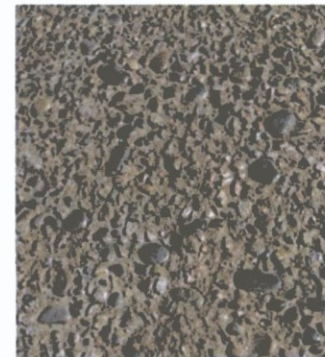
FL2 CONCRETE FLATWORK
