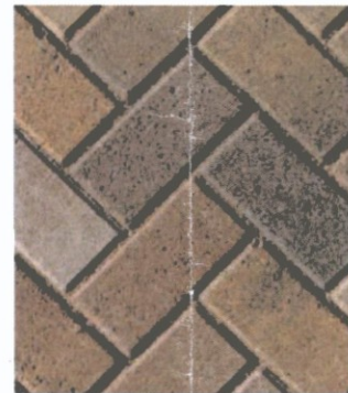
FL3 PRECAST CONCRETE PAVERS
