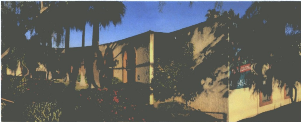
2 Existing North West Corner
