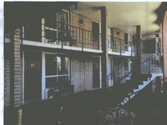
3 Existing North Elevation Interior
