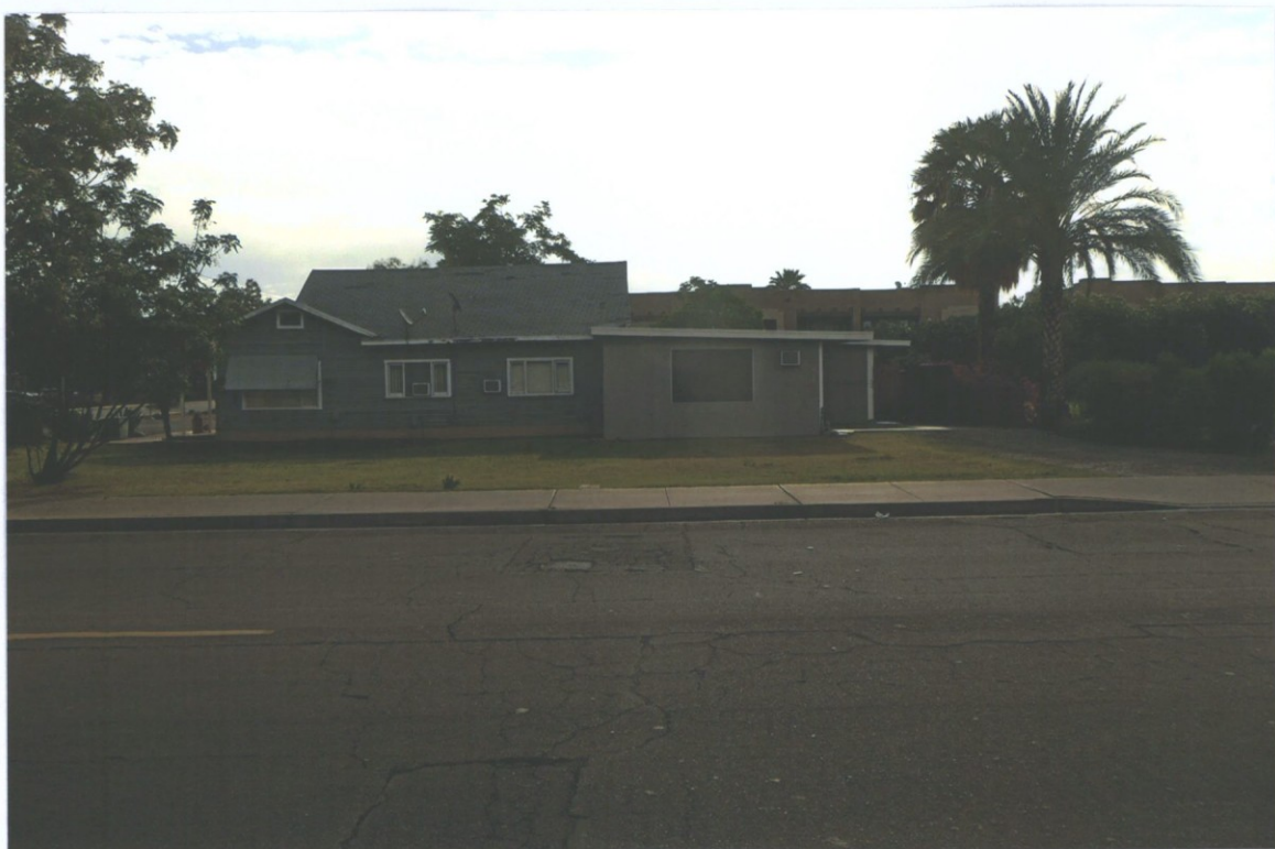
East side looking west
