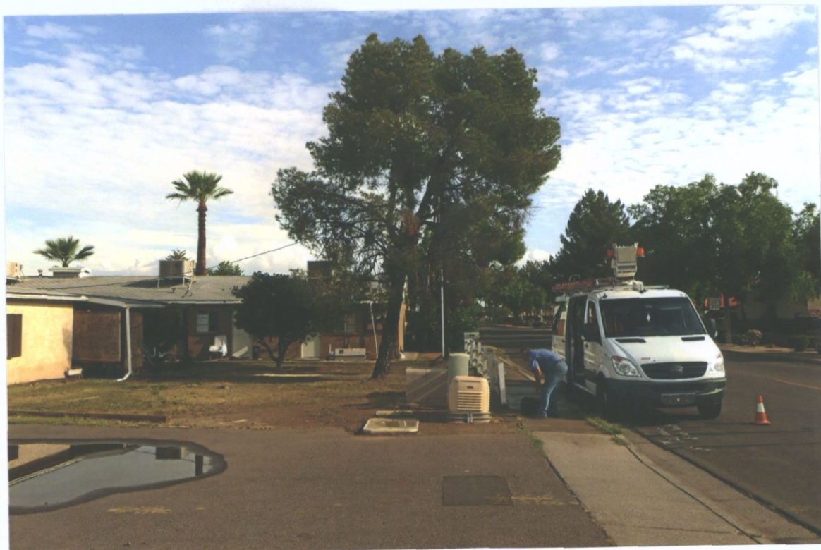
Northeast corner looking north
