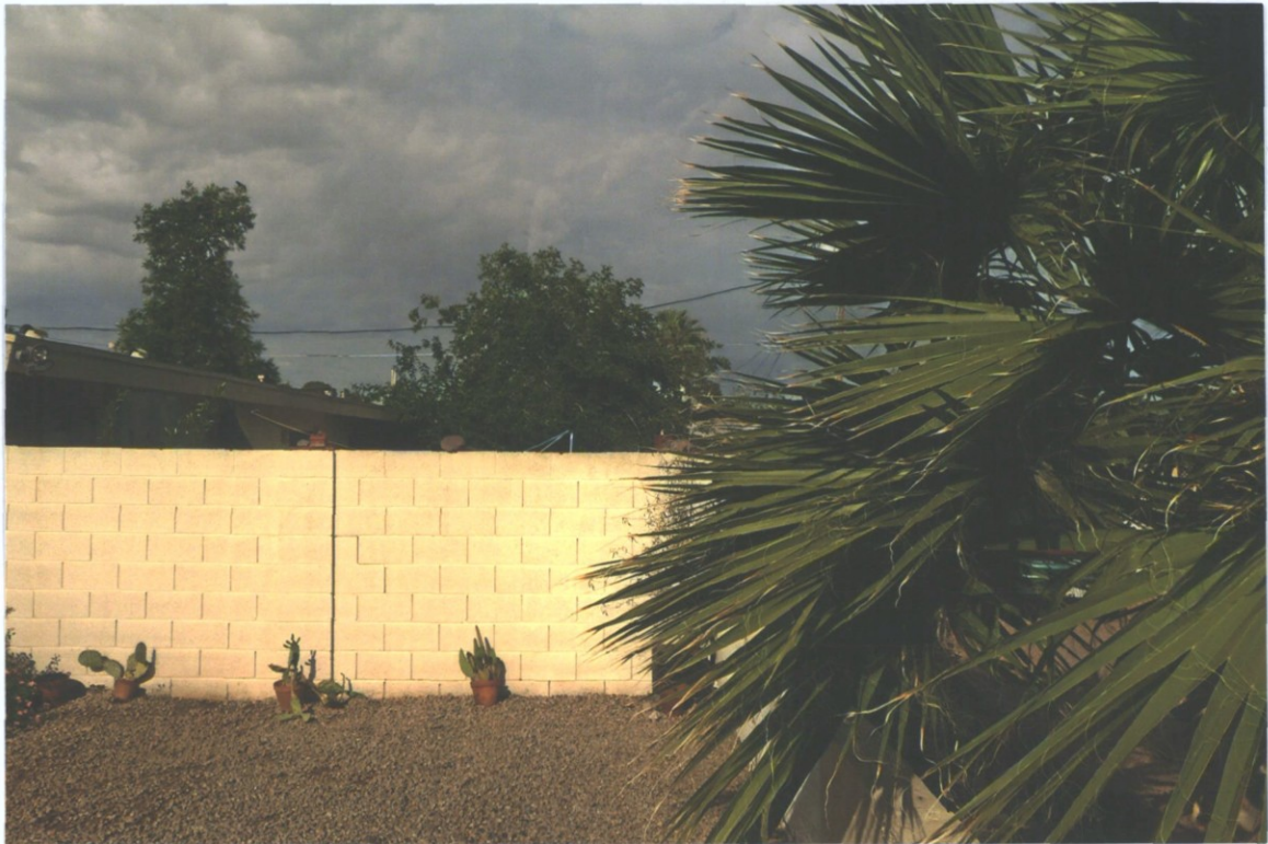
Southeast corner looking west
