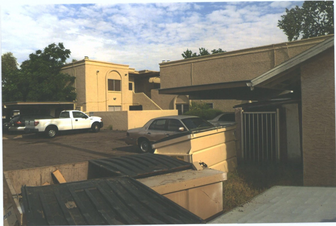
Northwest corner looking northwest
