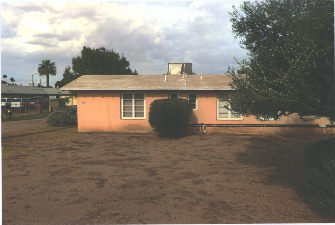
East side looking west
