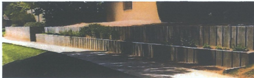
Existing common area greenway wall
