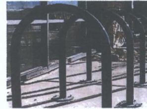
Multiple inverted racks shall be mounted in line and parallel as shown.
