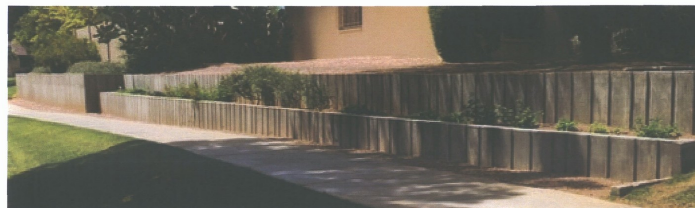
Existing common area greenway wall
