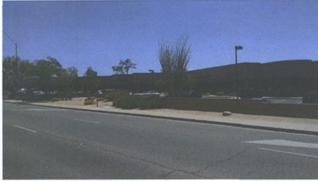
BUILDING 15425 - EXISTING CONDITION
