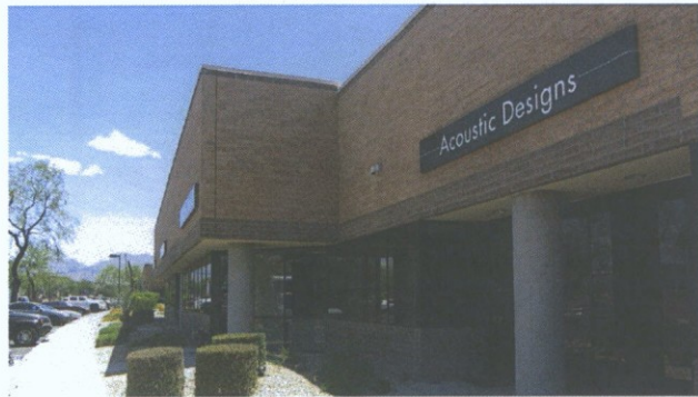
BUILDING 15475 - EXISTING CONDITION
