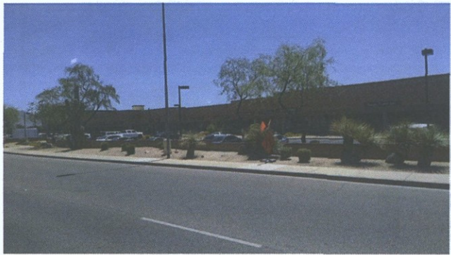
BUILDING 15425 - EXISTING CONDITION
