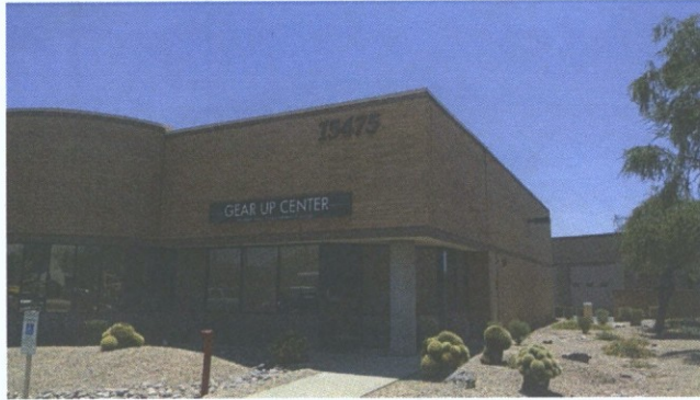
BUILDING 15475 - EXISTING CONDITION
