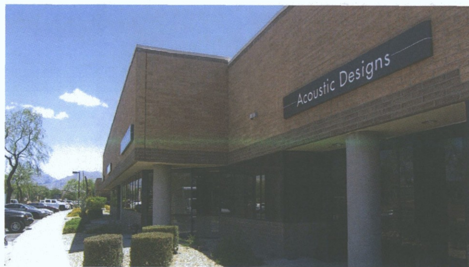
BUILDING 15475 - EXISTING CONDITION
