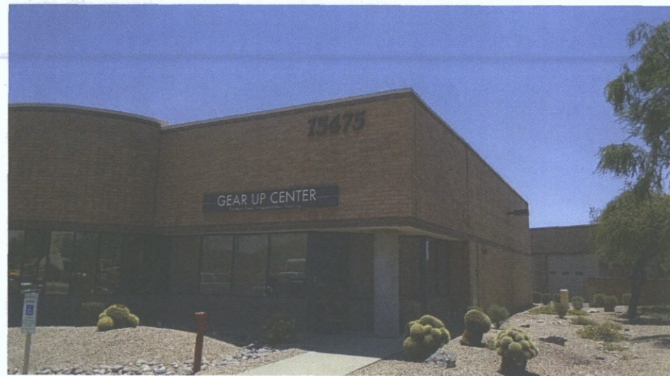
BUILDING 15475 - EXISTING CONDITION
