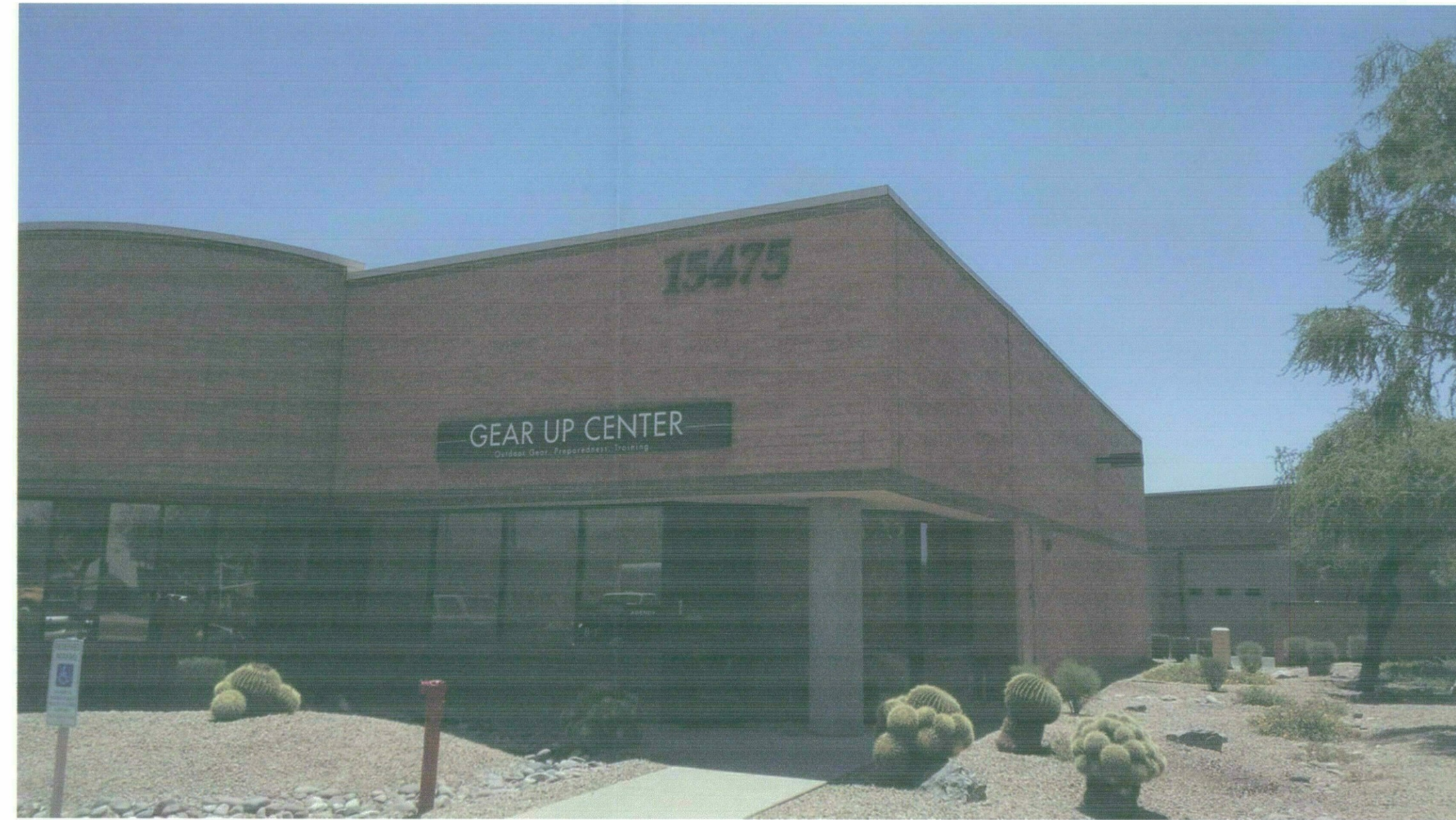
BUILDING 15475 - EXISTING CONDITION
