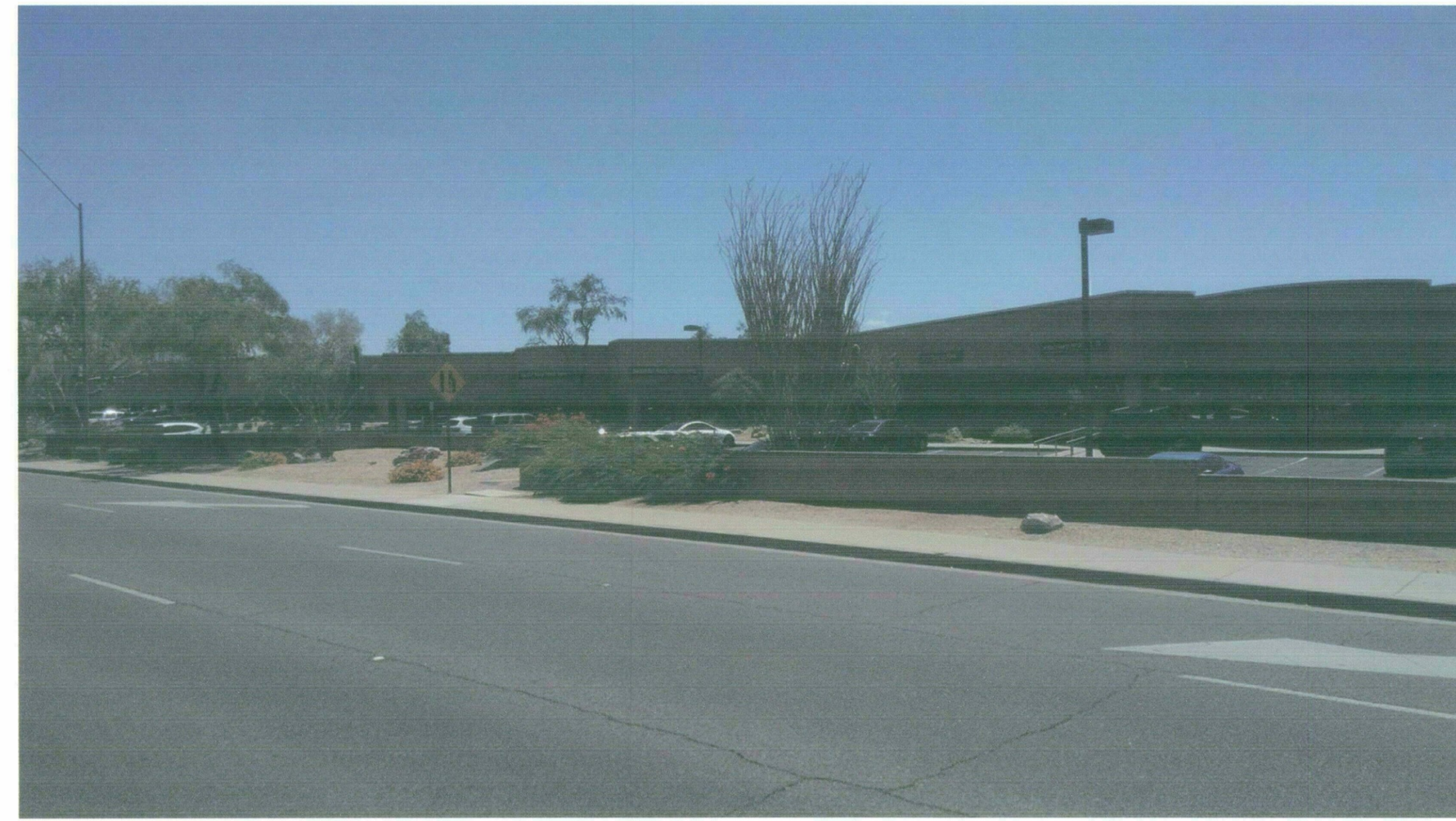
BUILDING 15425 - EXISTING CONDITION
