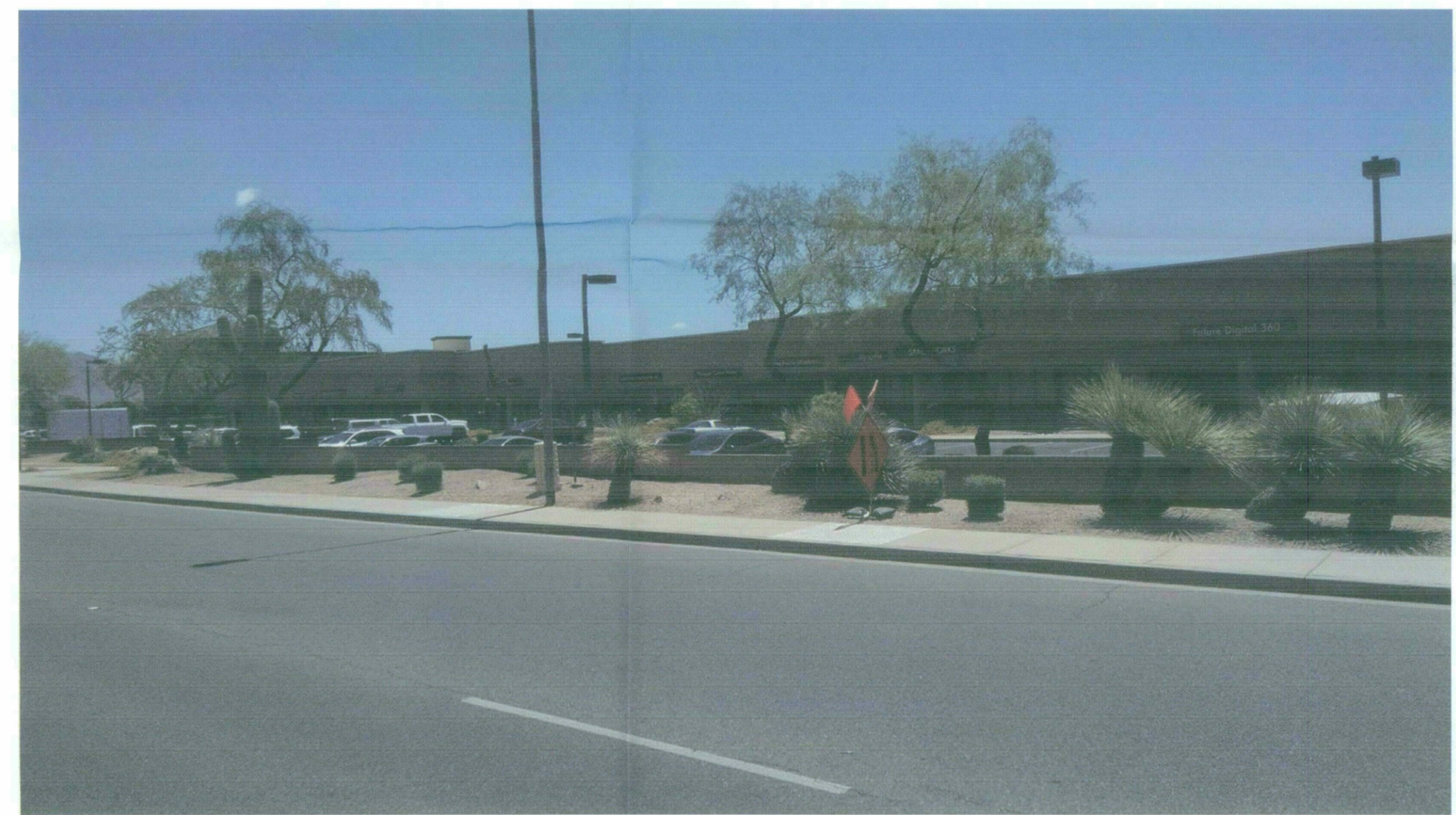
BUILDING 15425 - EXISTING CONDITION
