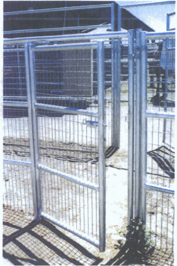
Close up of open interior service gate, 4 ft. wide, 8 ft. tall.
