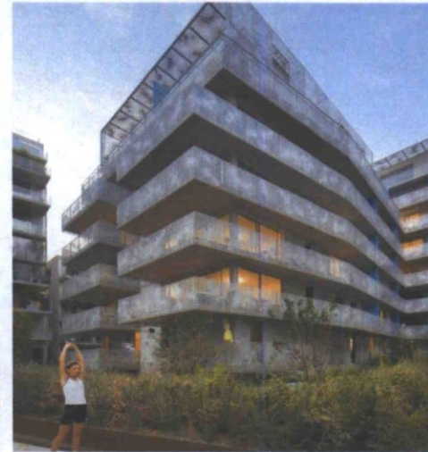
Apartment Complex, Rives de Seine, France
