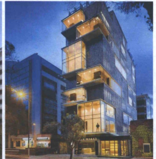
Apartment Complex, Paris, France
