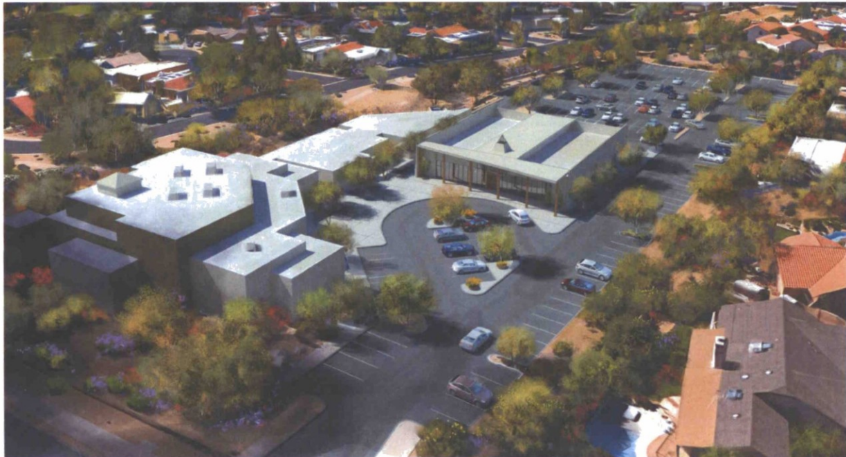
VIEW LOOKING SOUTHEAST FROM SHEA
