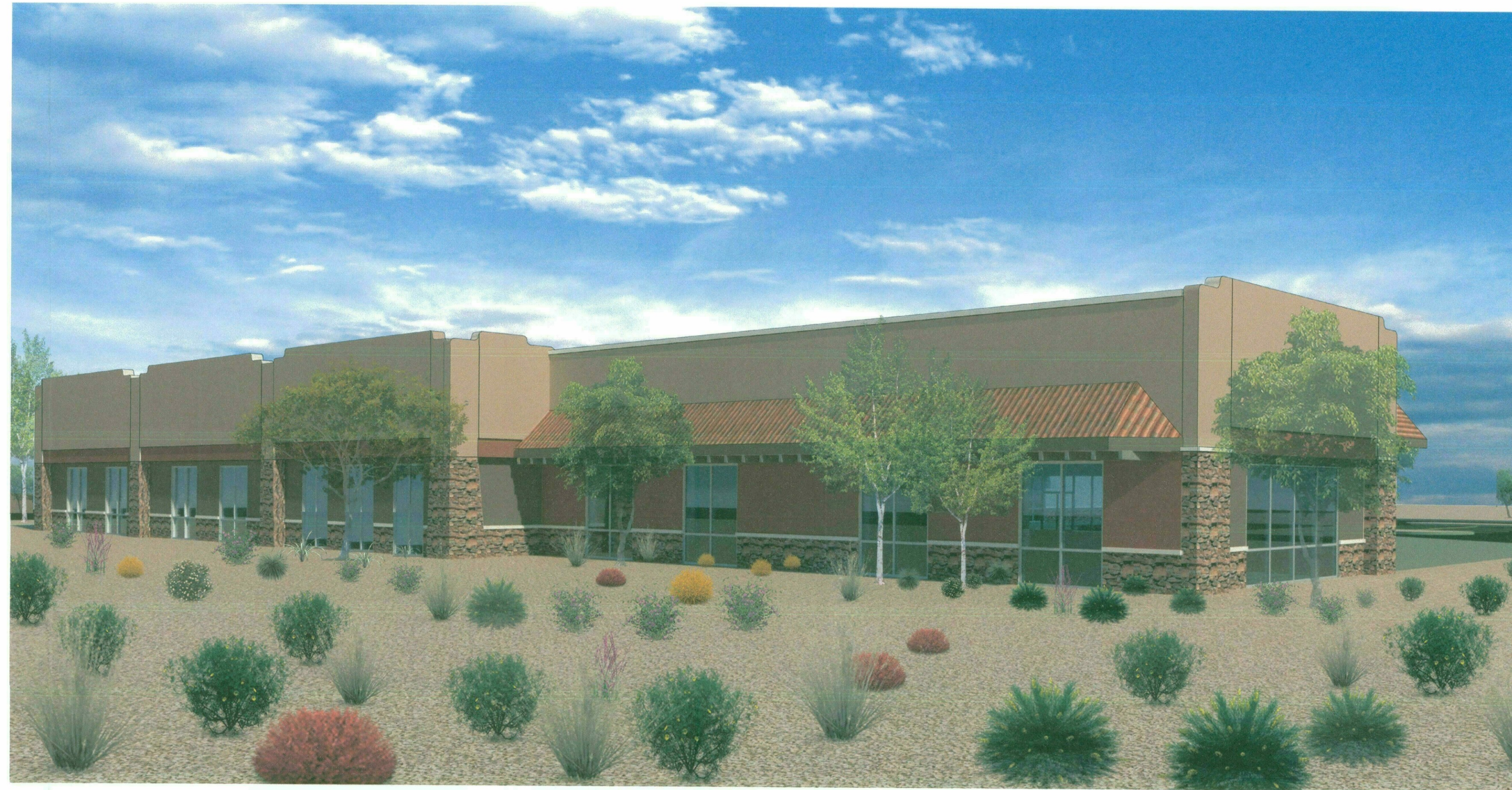
VIEW LOOKING SOUTH EAST ON 116TH & SHEA
