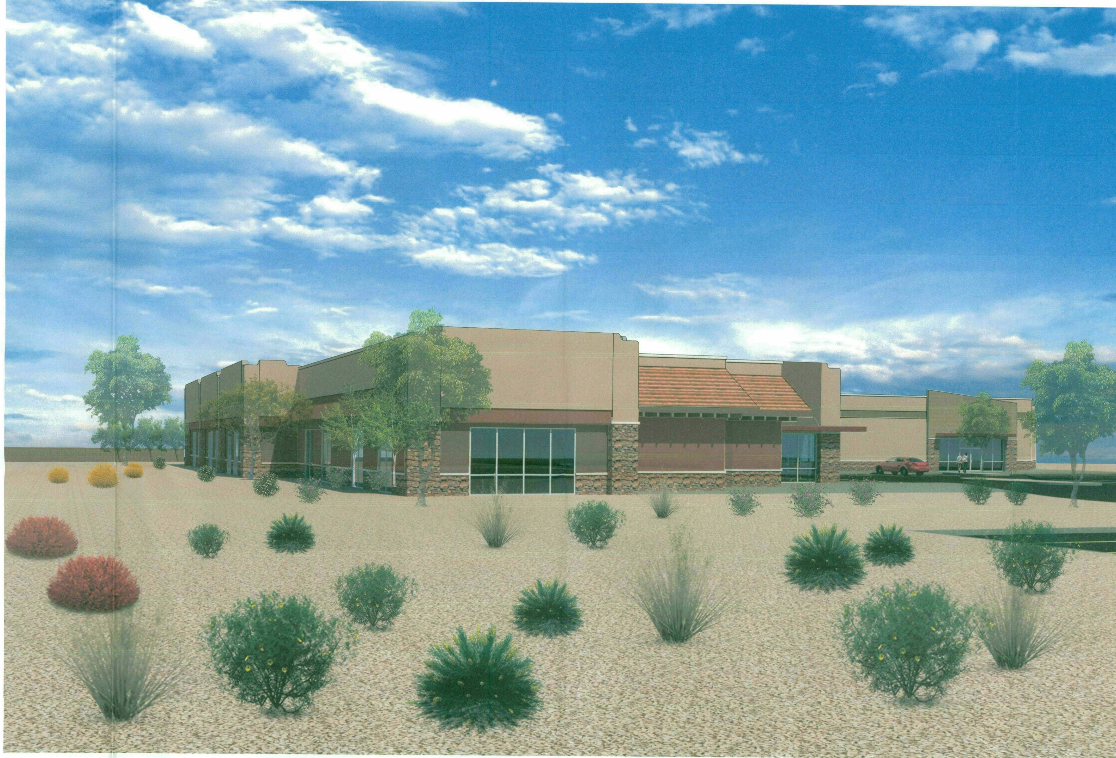
VIEW LOOKING SOUTH EAST ON 116TH & SHEA
