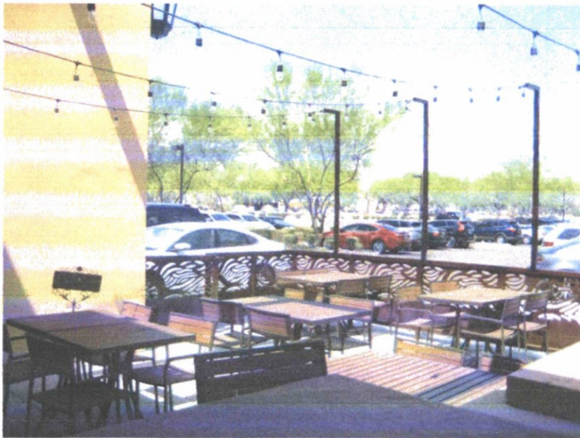
Photo 2 Existing open area for covered patio
