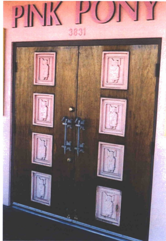
Entry doors with iron hardware
