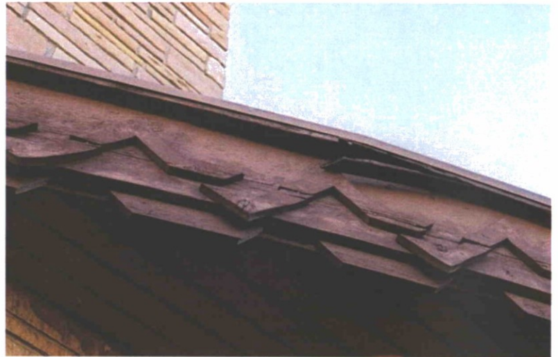
Canopy fascia and trim
