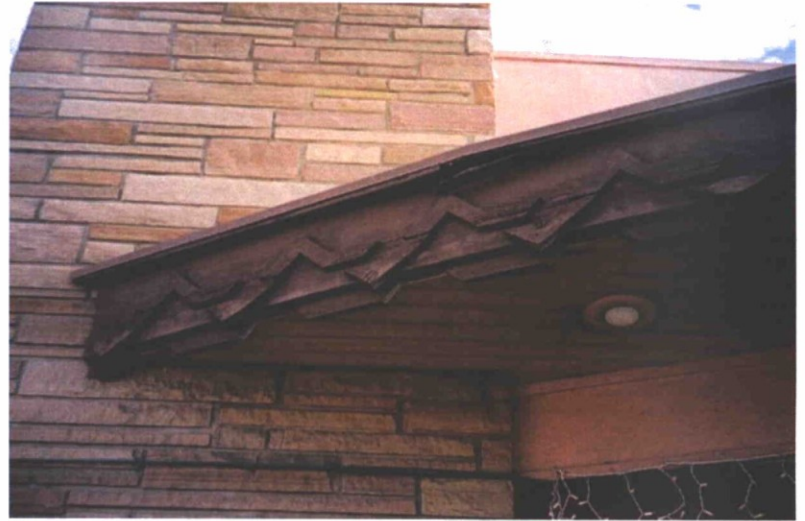
Wood fascia board trim and recessed light underneath canopy
