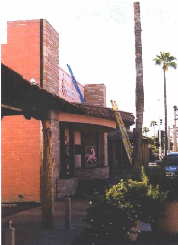
Looking south at corner elements and parapets
