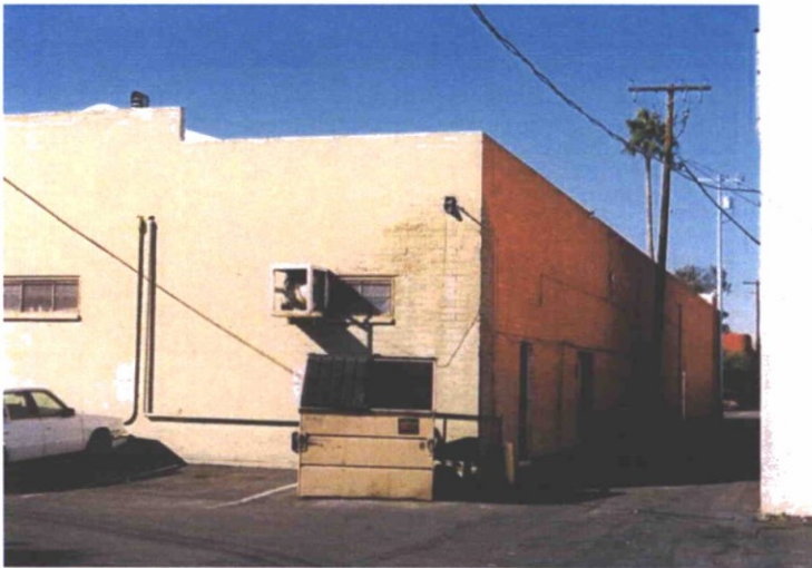
Rear and alley side elevations showing massing
