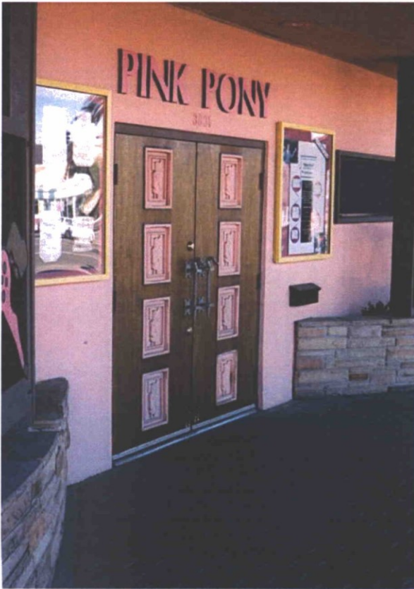
Stucco wall around recessed entry
