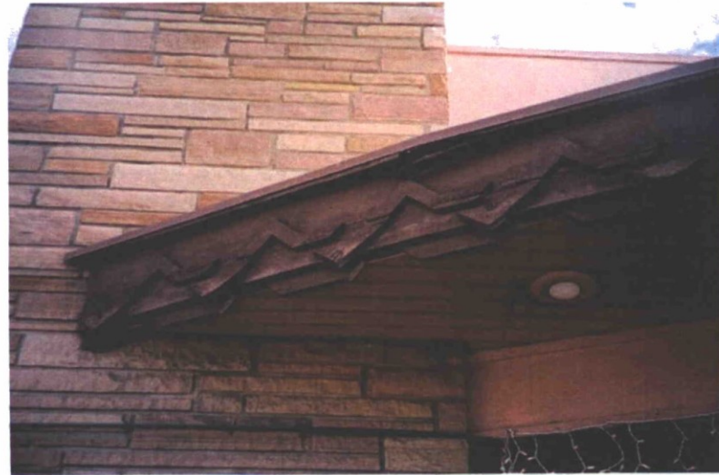
Wood fascia board trim and recessed light underneath canopy
