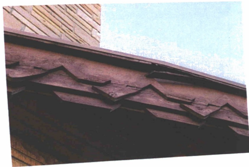
Canopy fascia and trim
