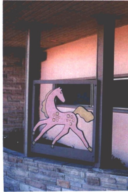
Wooden posts supporting canopy and horizontal window
