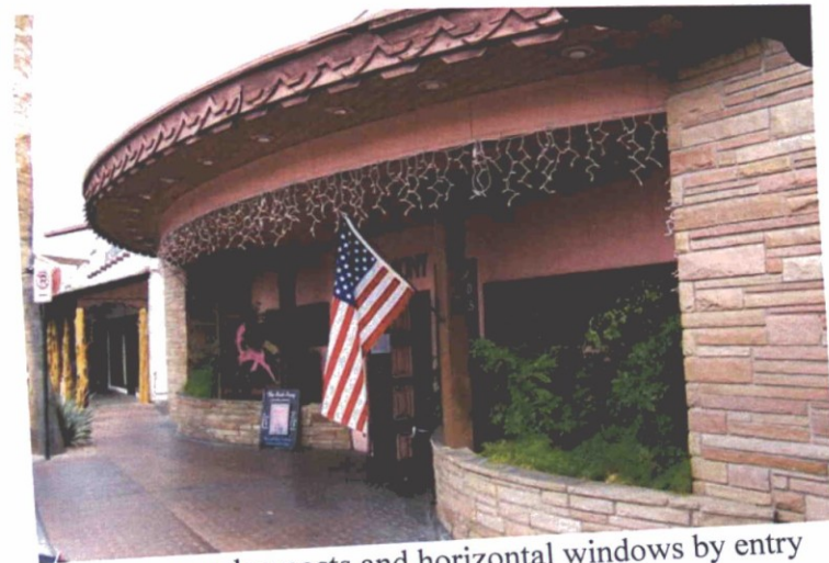
Wooden posts supporting canopy and horizontal window
