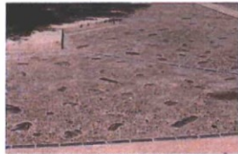
HANDSEEDED CONCRETE ACCENT PAVING
