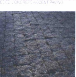
Handseeded concrete accent paving
