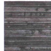
BOARD FORM CONCRETE
