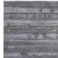
BOARD FORM CONCRETE
