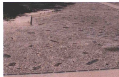
HANDSEEDED CONCRETE ACCENT PAVING
