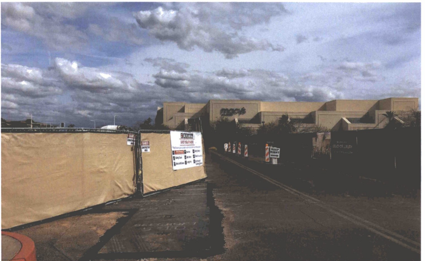
#6 east looking east
