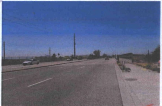
West along Shea Boulevard
