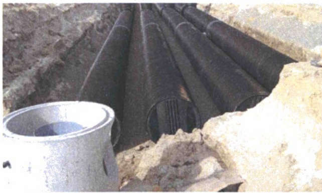
CDS pretreats a rainwater harvesting cistern.
