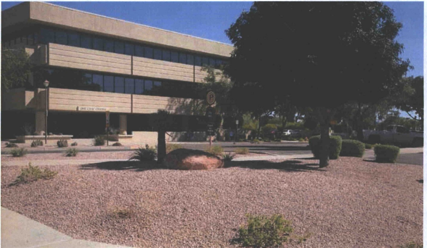
Looking North East
