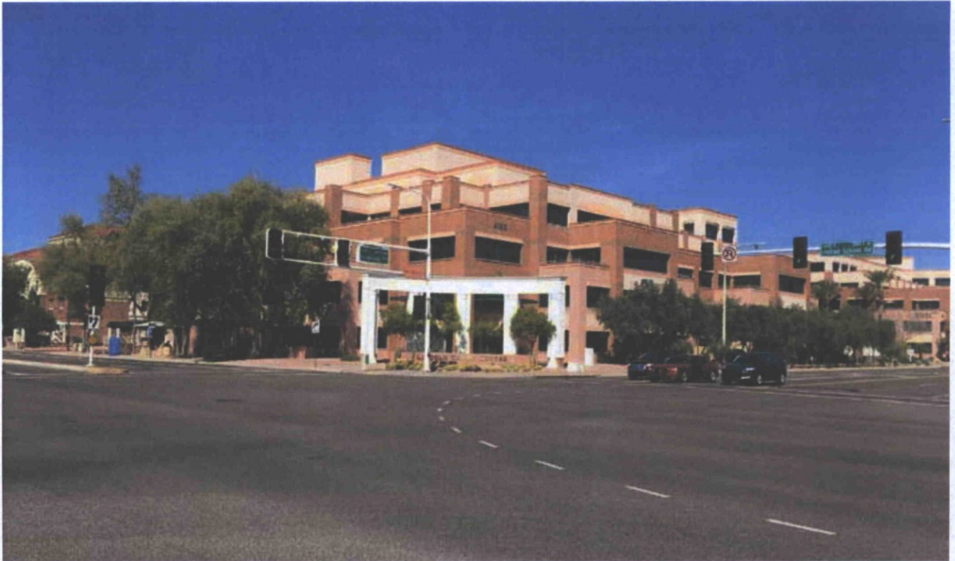
Looking North West
