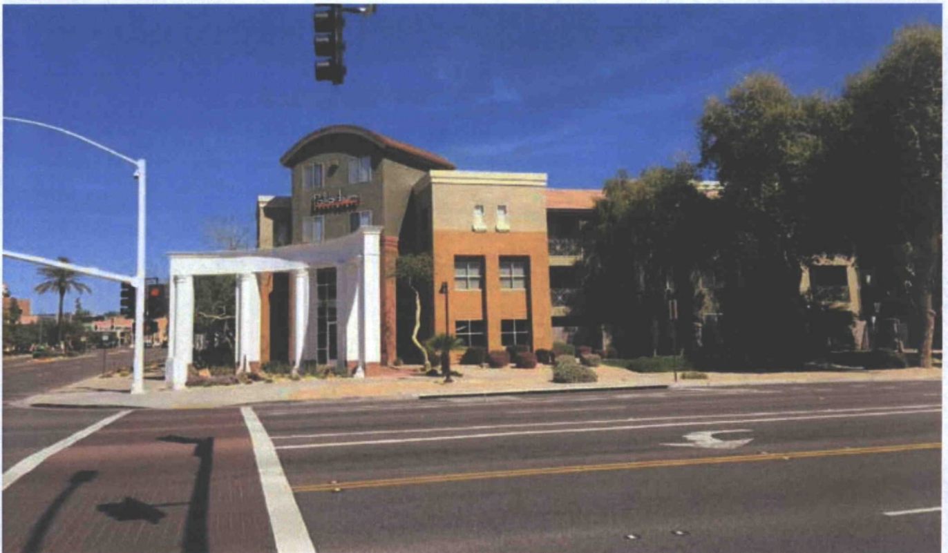
Looking North East
