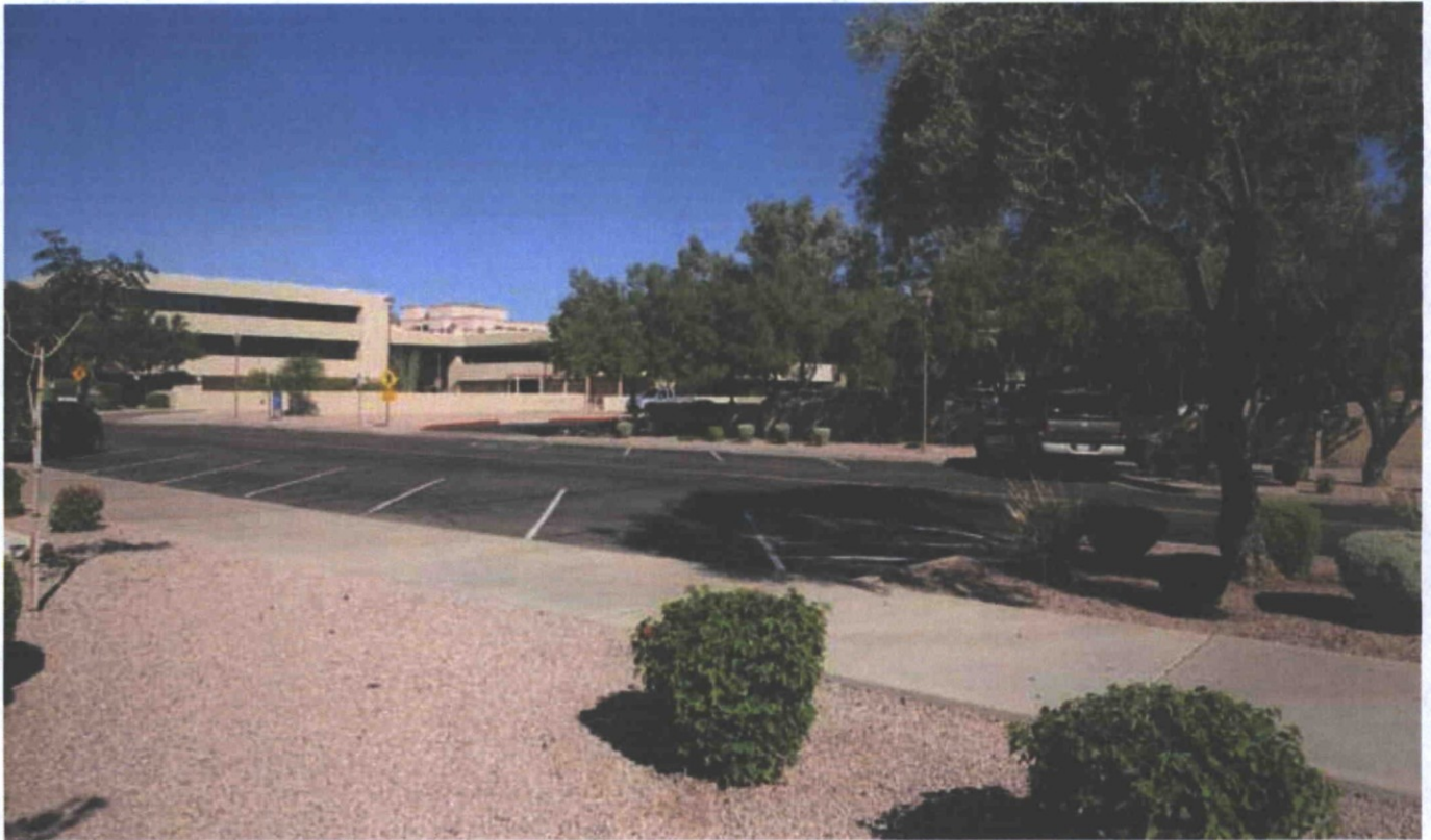
Looking North West
