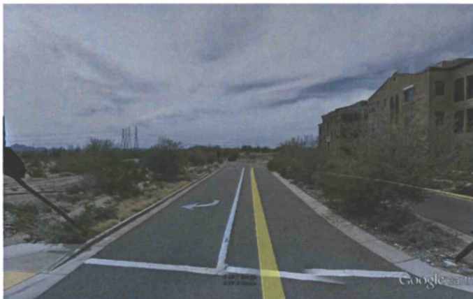
NEC looking west
