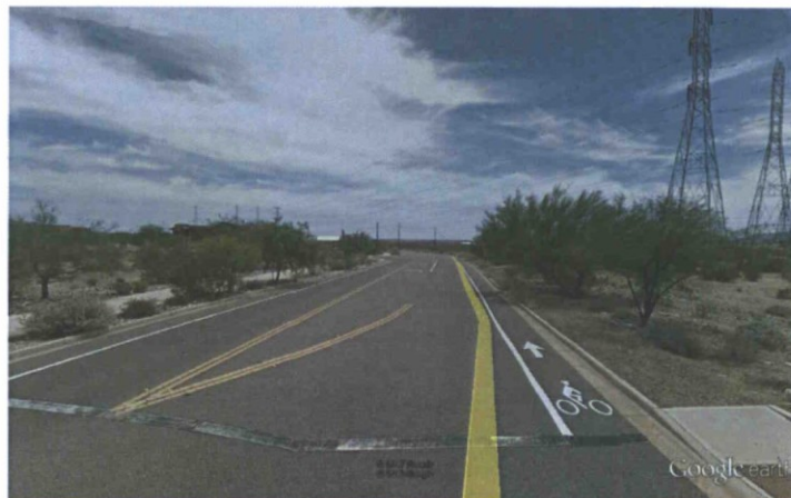
SEC looking south
