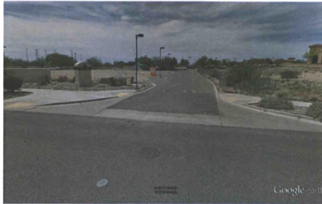
NWC looking west
