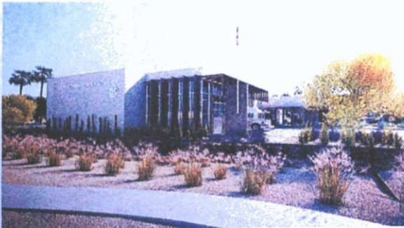
CITY OF SCOTTSDALE FIRE STATION #603 Exterior Building Color & Material Sample Board 1 of 2
