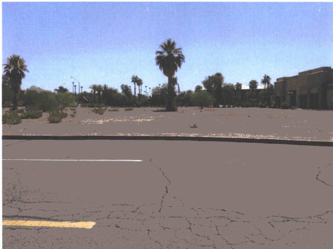
Photograph 14 (from west edge of site, view to east)
