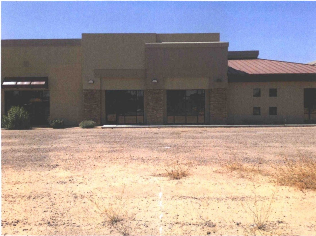
Photograph 11 (from south edge of site, view to south)
