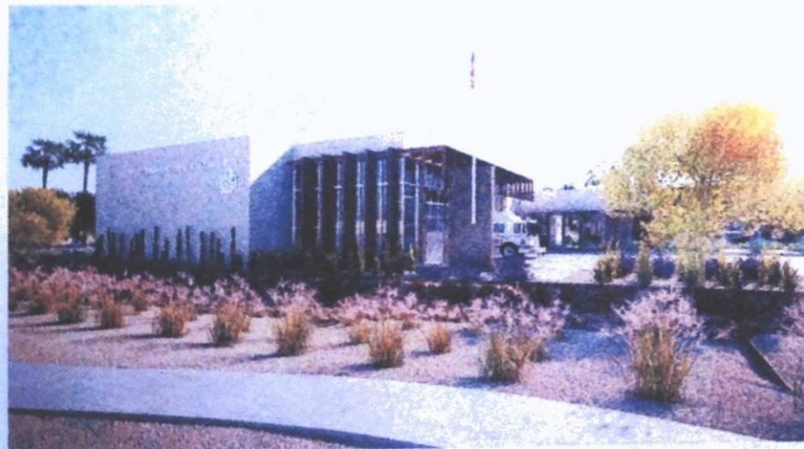
CITY OF SCOTTSDALE FIRE STATION #603 Exterior Building Color & Material Sample Board 1 of 2
