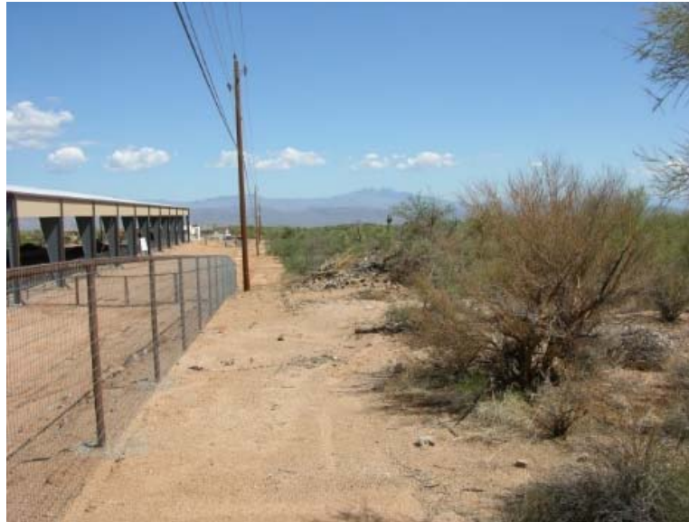
AT&T Mobility 136 TH Street & Rio Verde Drive 12kV Distribution Pole
