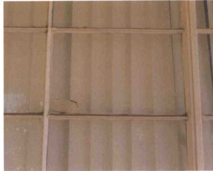
12. Window 5 cracks in panes facing South
