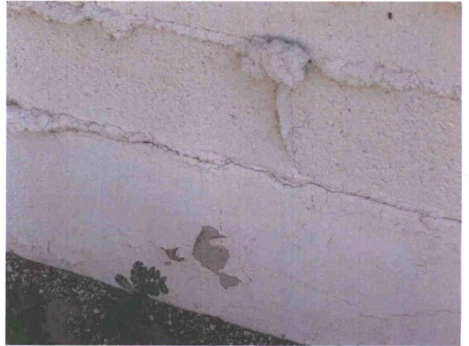
6. Peeling paint on brick plus weeping mortar facing North
