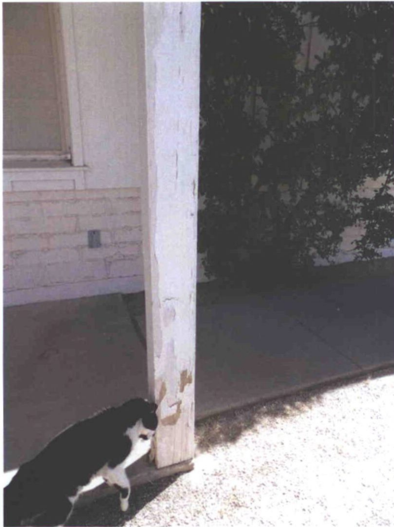
9. Peeling paint on post facing North.
