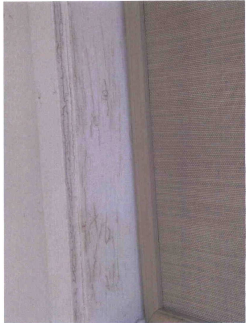
8. Peeling paint on window trim. Window 1 faces North; trim faces West
