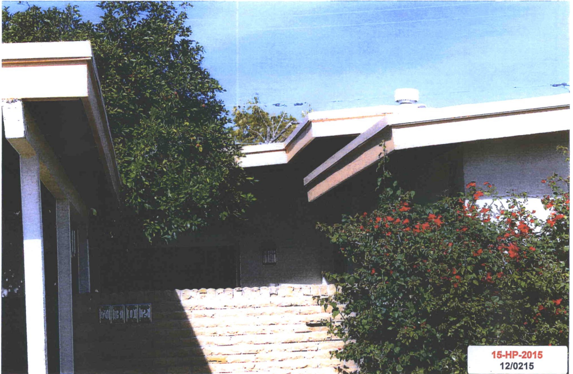
Town & Country Haver Home showing proper drip edge.
