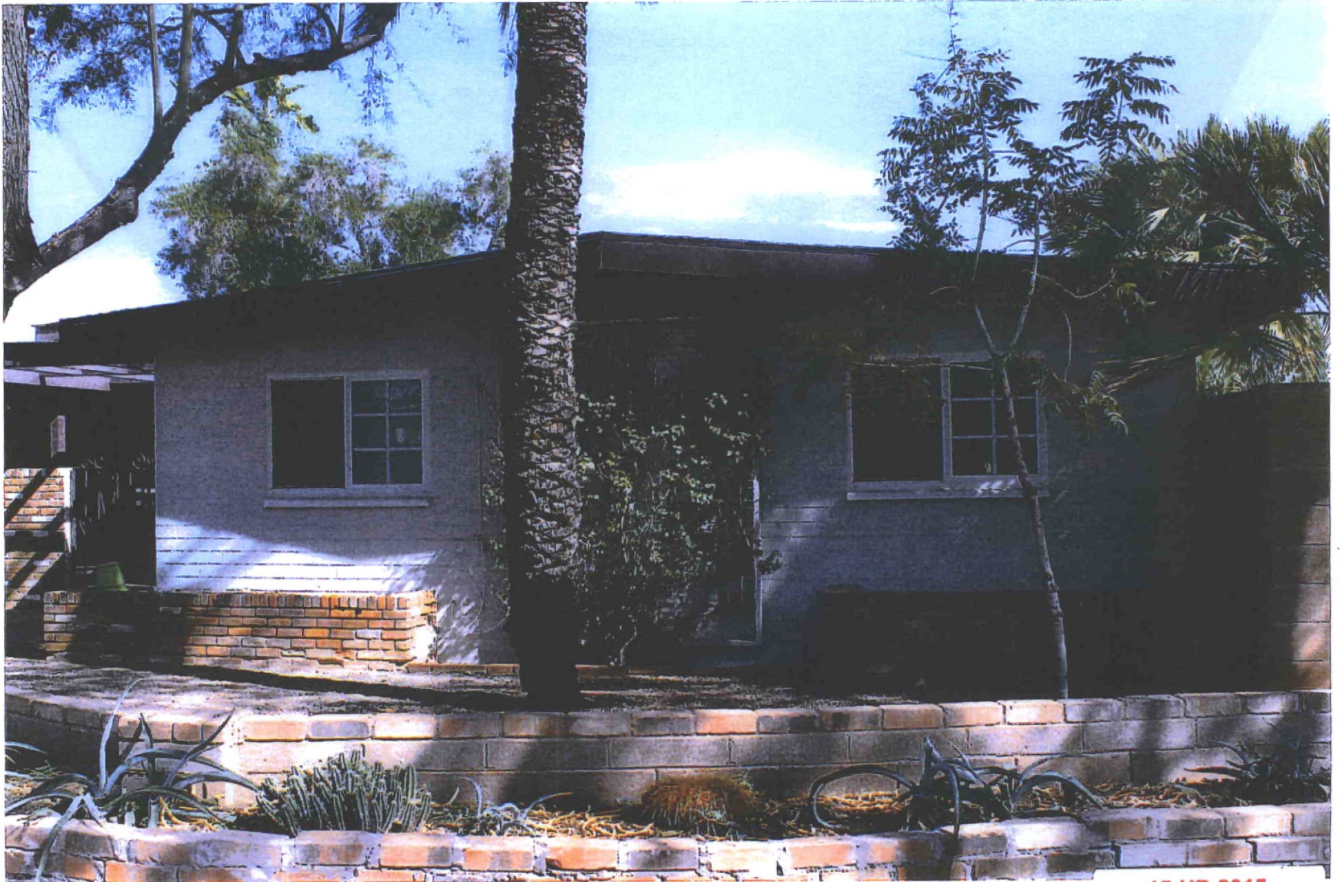
View of property from street. (72nd Place)
