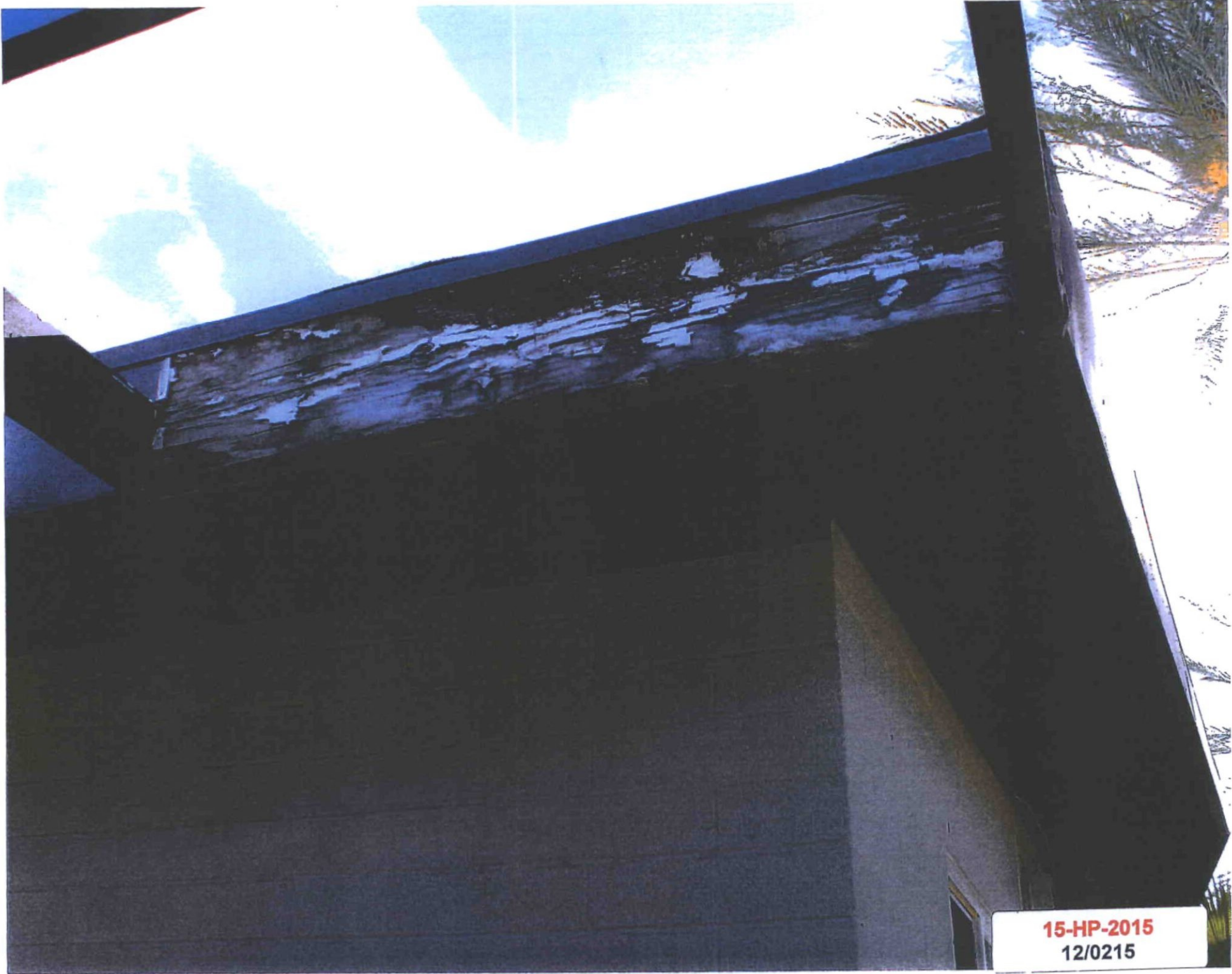
Damage: fascia - open framing (walk-way)
