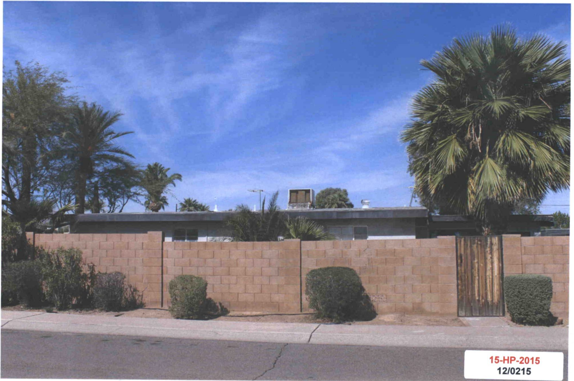
Side view of property, from Monte Vista. Project will remove deteriorated Swamp Cooler.
