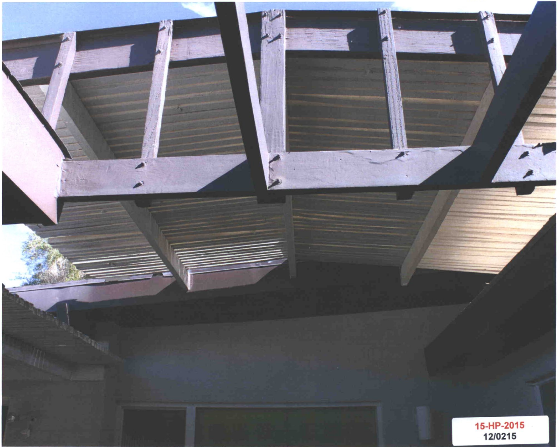
wood framing above walk way (Remove, restore to original.)
