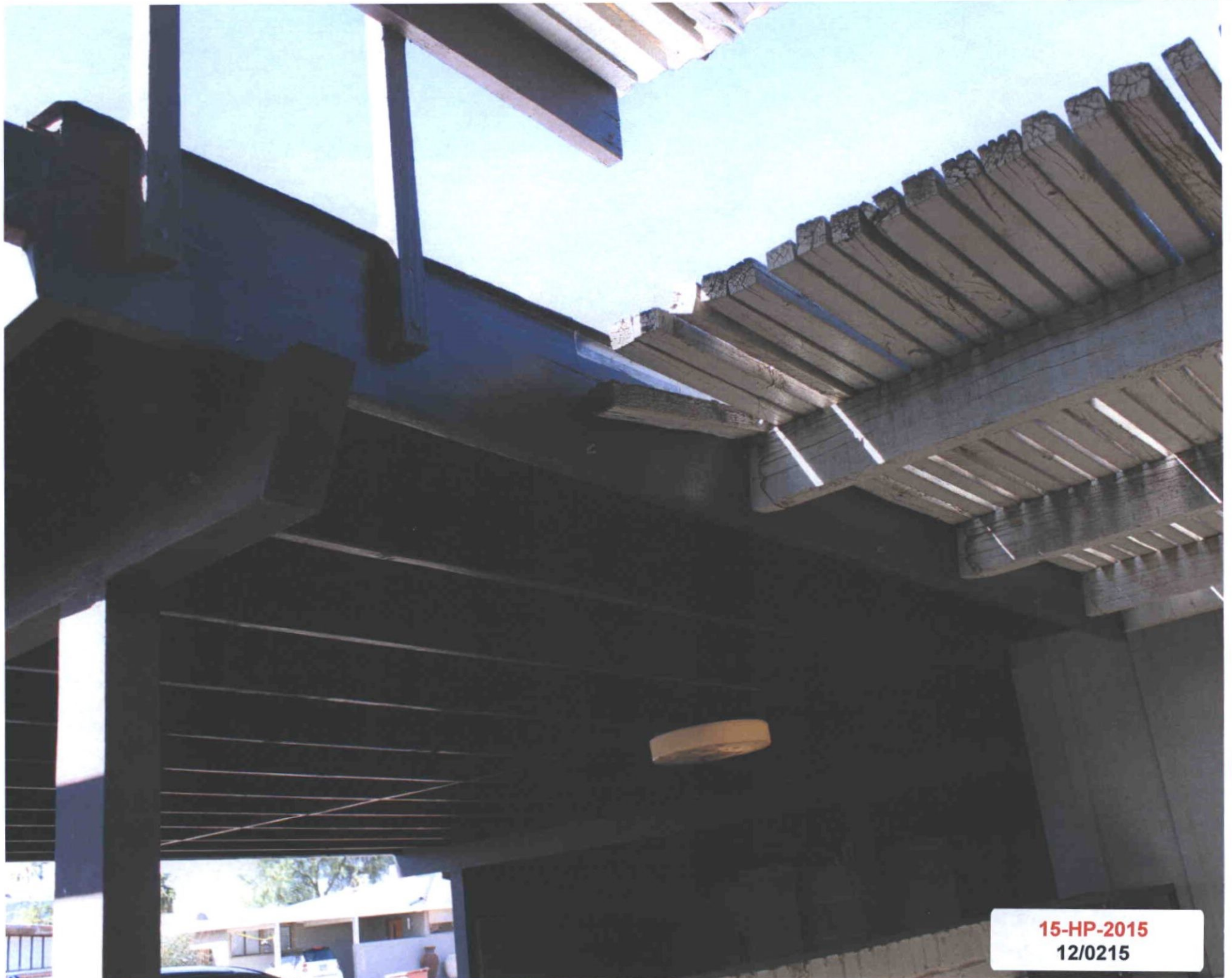
Damage: Wood framing, car port beam
