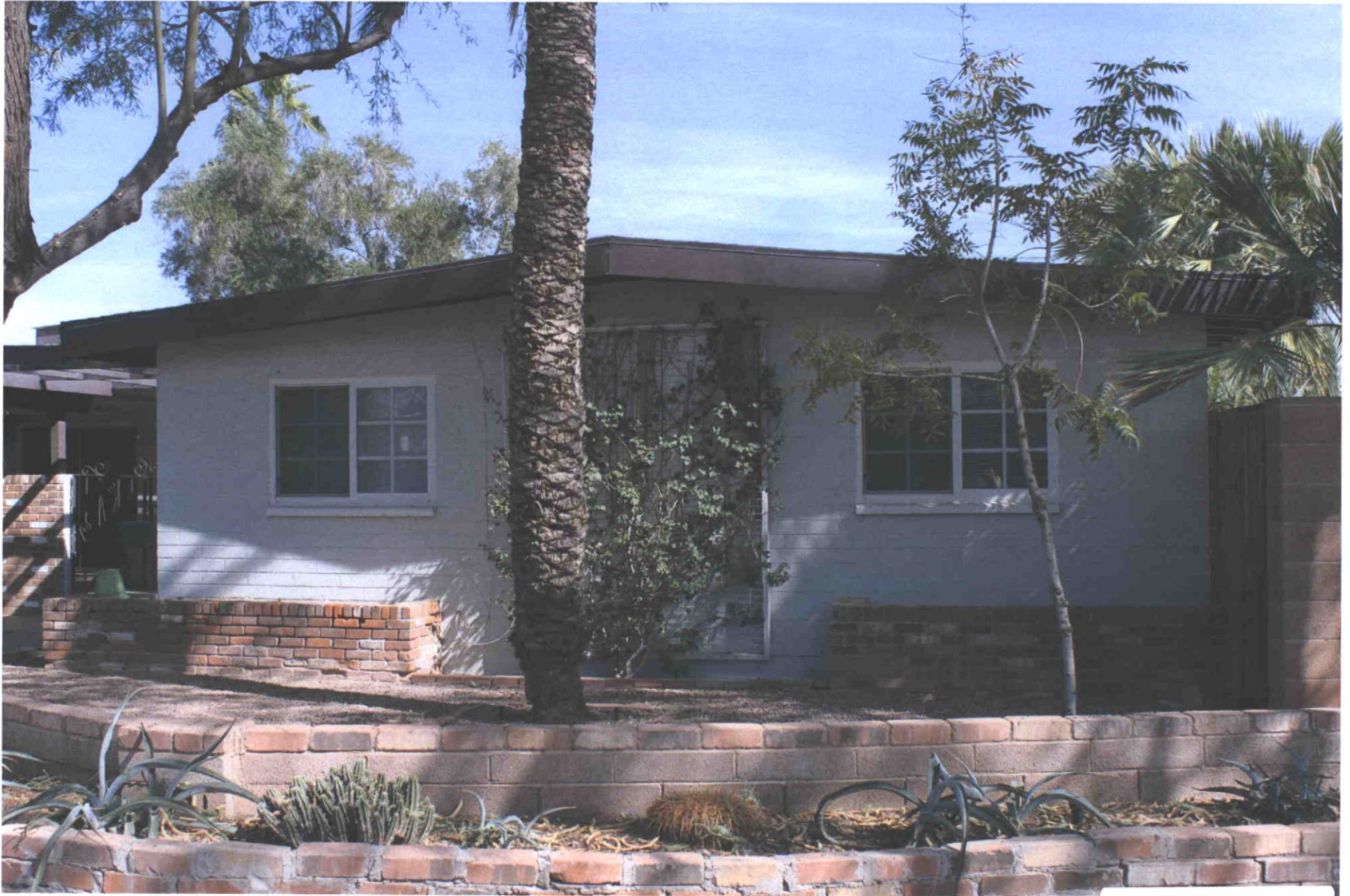
View of property from street. (72nd Place)
